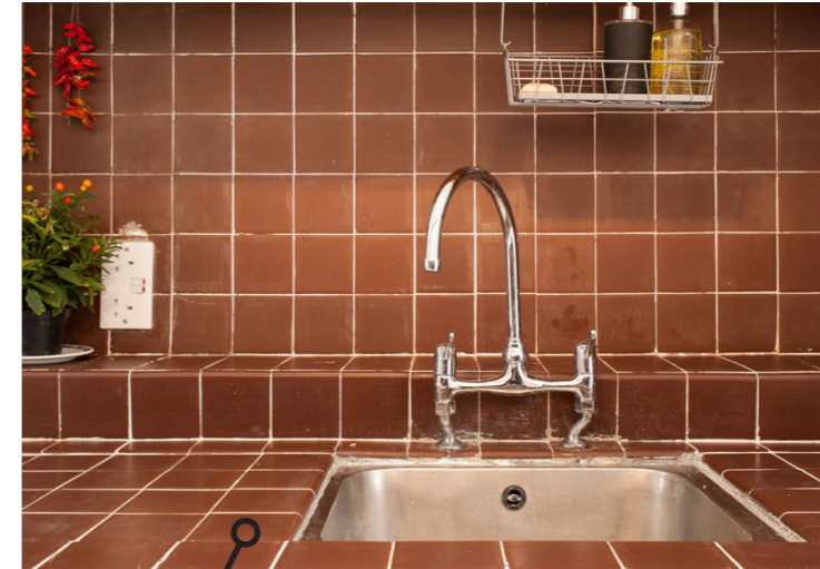
Original kitchen tiles
