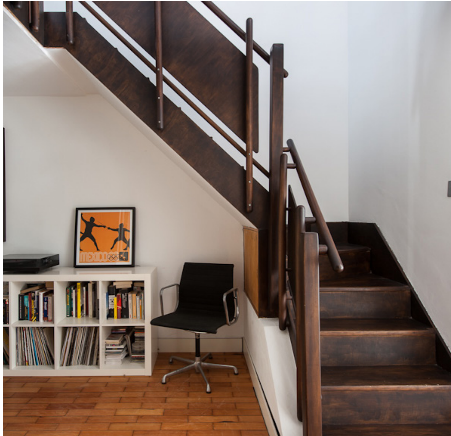
Current stair stain
