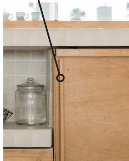
Original kitchen doors
