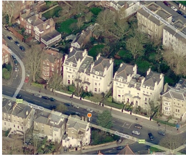
Fig. 2 Ariel View from West
