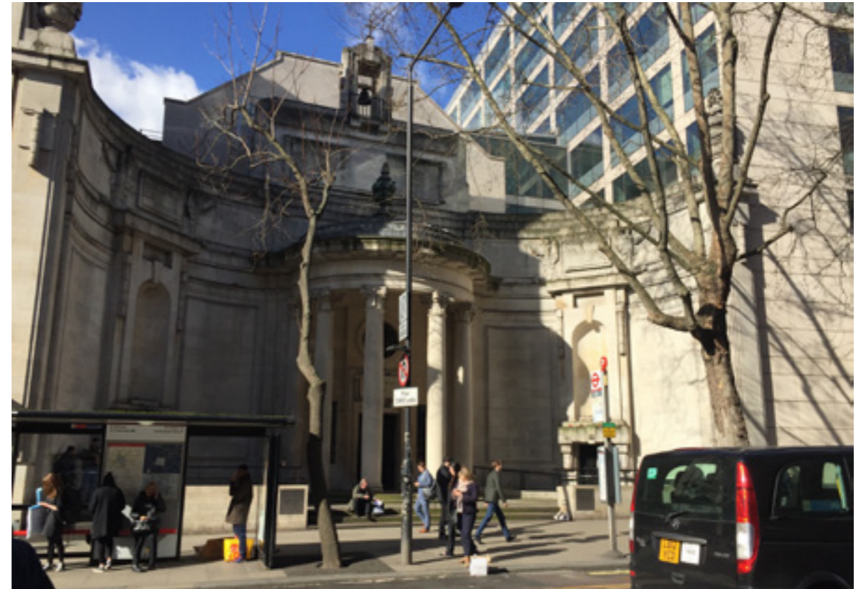
View looking west at the retained facade of The Holy Trinity Church which is now the entrance to the modern office building of Aviation House. The remainder of the church has been demolished.
