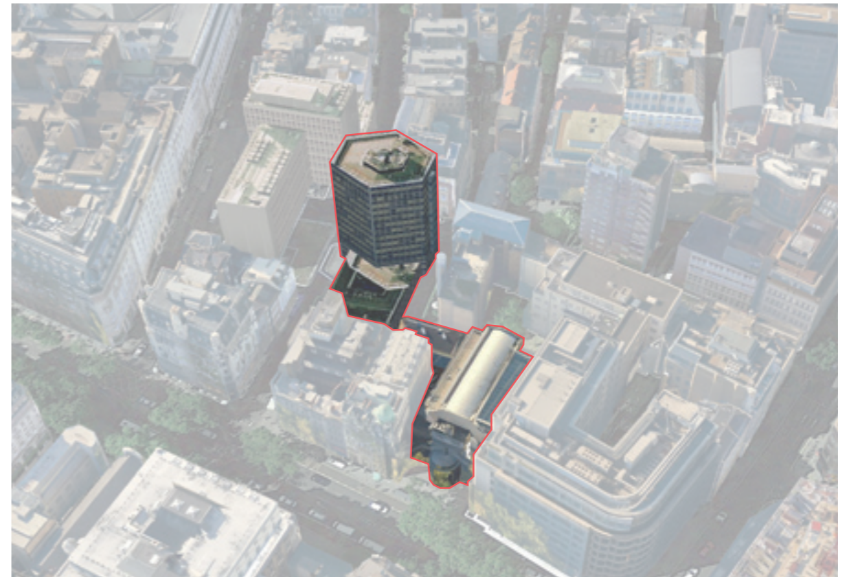
Aerial view of the site looking west.
