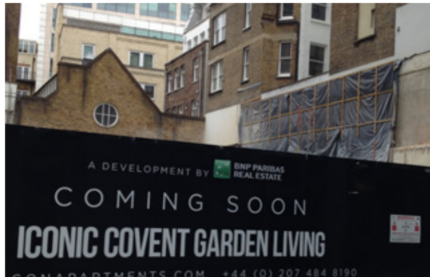
Temporary view of the window from Parker Street following demolition. The approved replacement buildings will cover the window opening.
