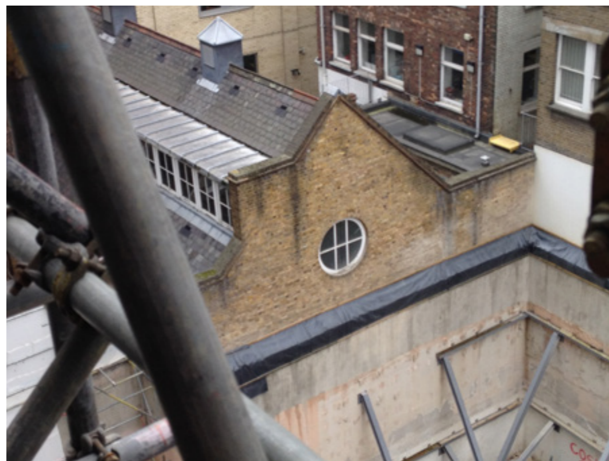
Existing Circular Window, as seen from neighbouring Parker Tower. (Currently undergoing development work).
