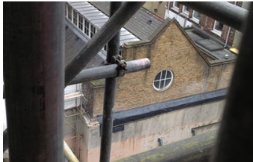
View of the window taken from the scaffold of Parker Tower.
