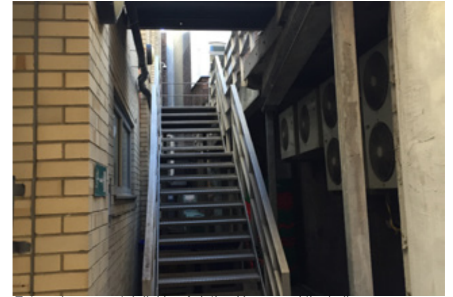
External access stair linking Aviation House and the hall.
