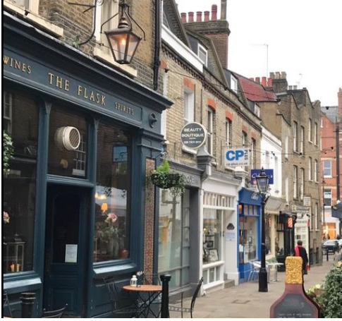
Fig 2 Flask Walk East side from north showing nos 6-12 (beyond the Flask pub), no 4 with tiled cheek of roof extension and no 2 with V parapet
