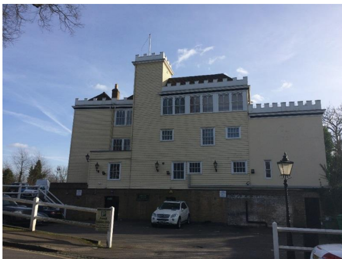
Figure 5.2 The assessment site overlooked by the adjacent building
