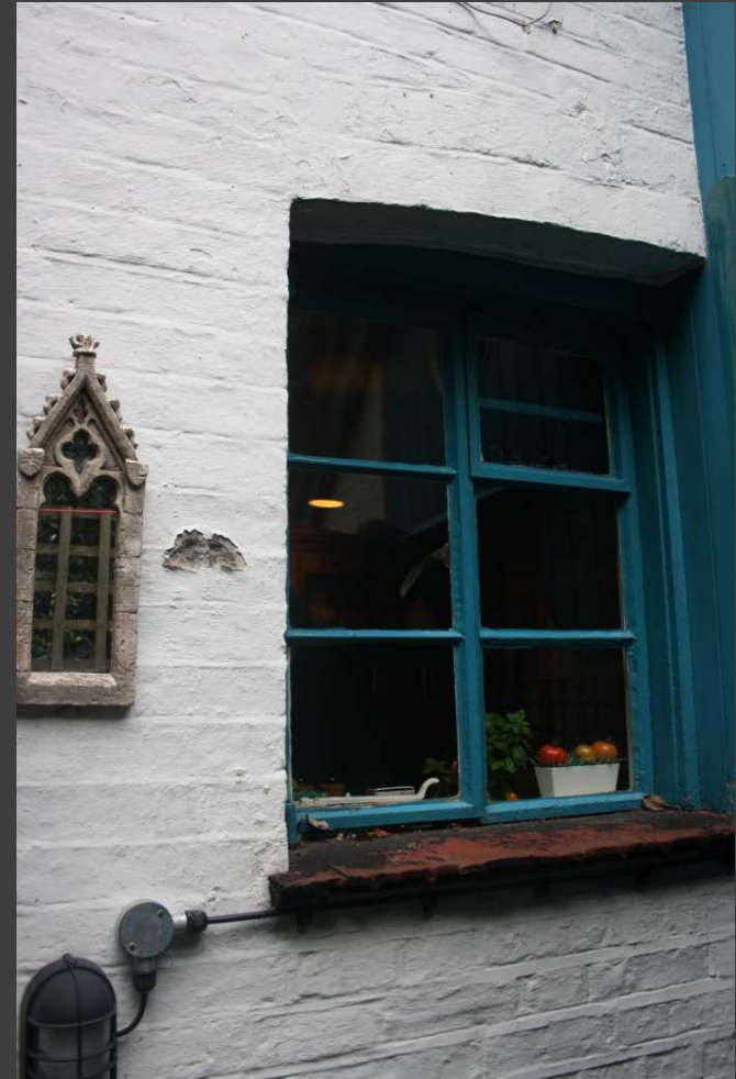
View of ground floor steel window to rear WG.05
