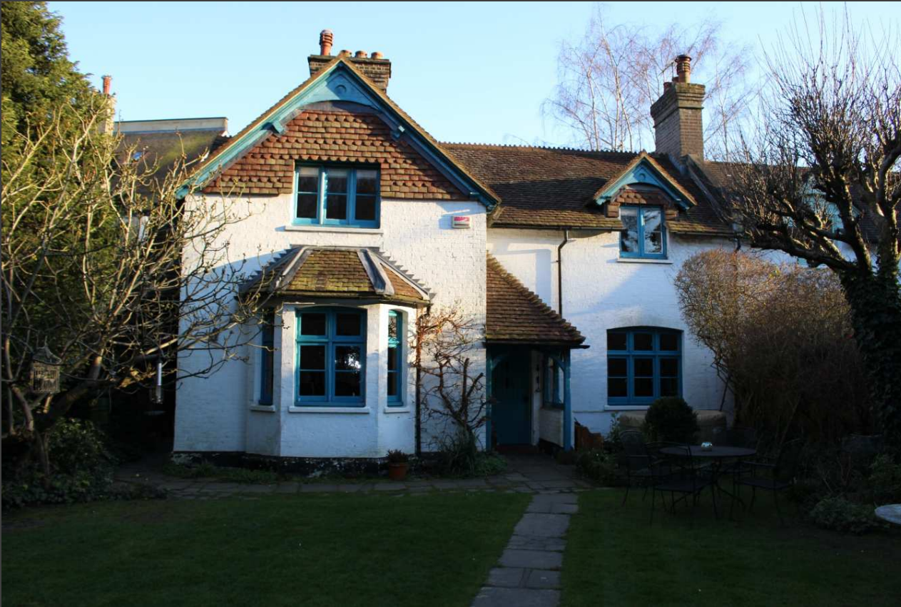
Existing northwest facing view of Vivary Cottage - garden and entrance elevation
