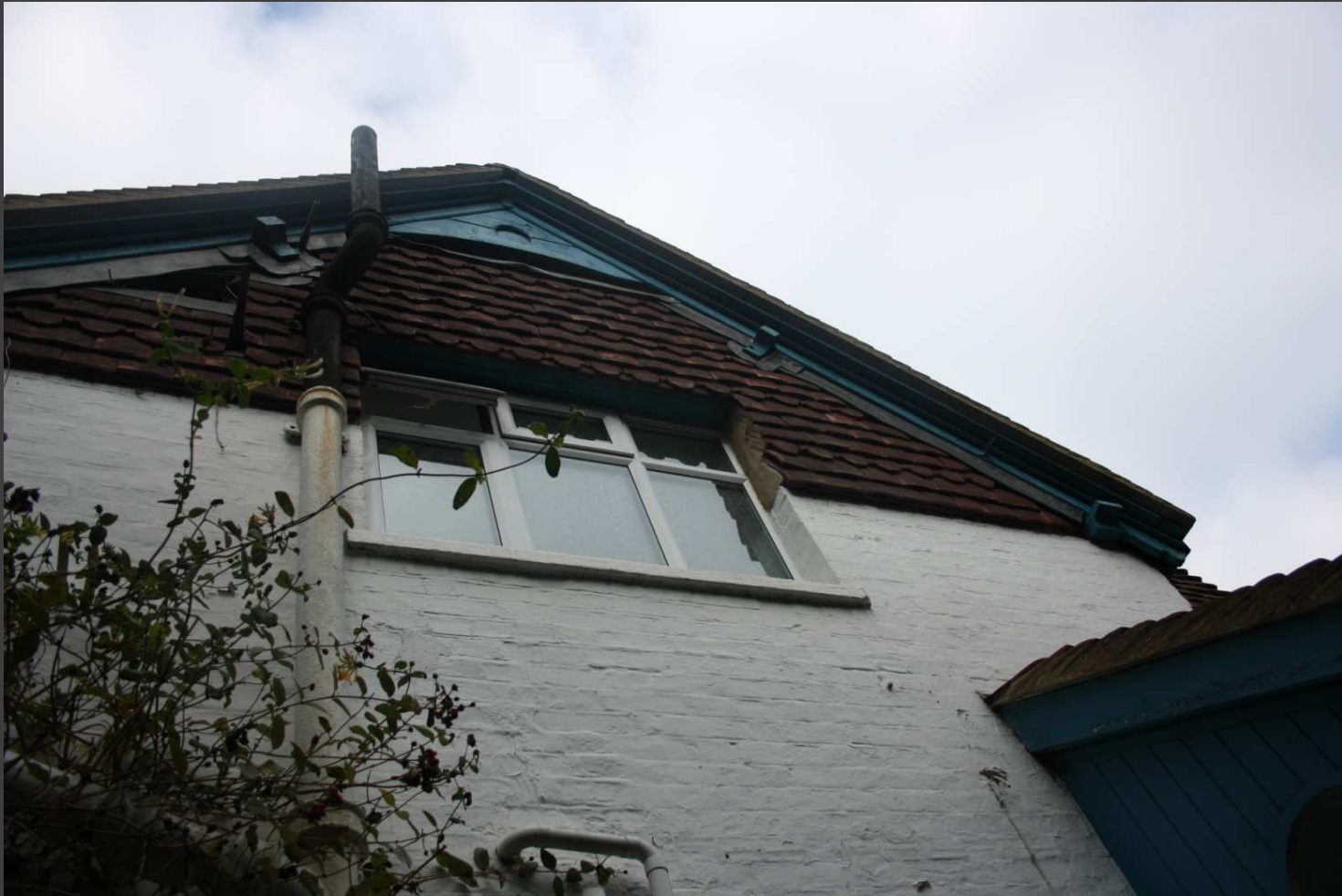
View of double glazed upvc window to rear W1.03
