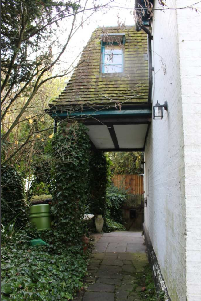
View of side extension showing steel window W1.05
