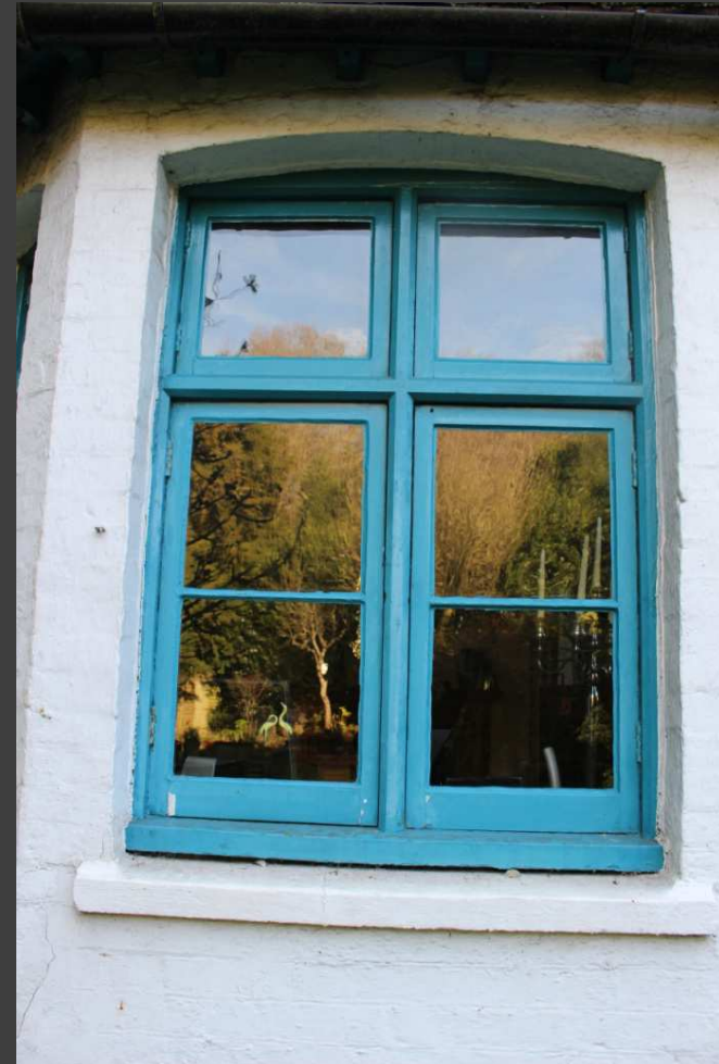
View of typical timber casement window, considered to be original.
