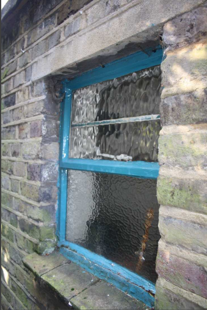
View of ground floor steel window to rear WG.02
