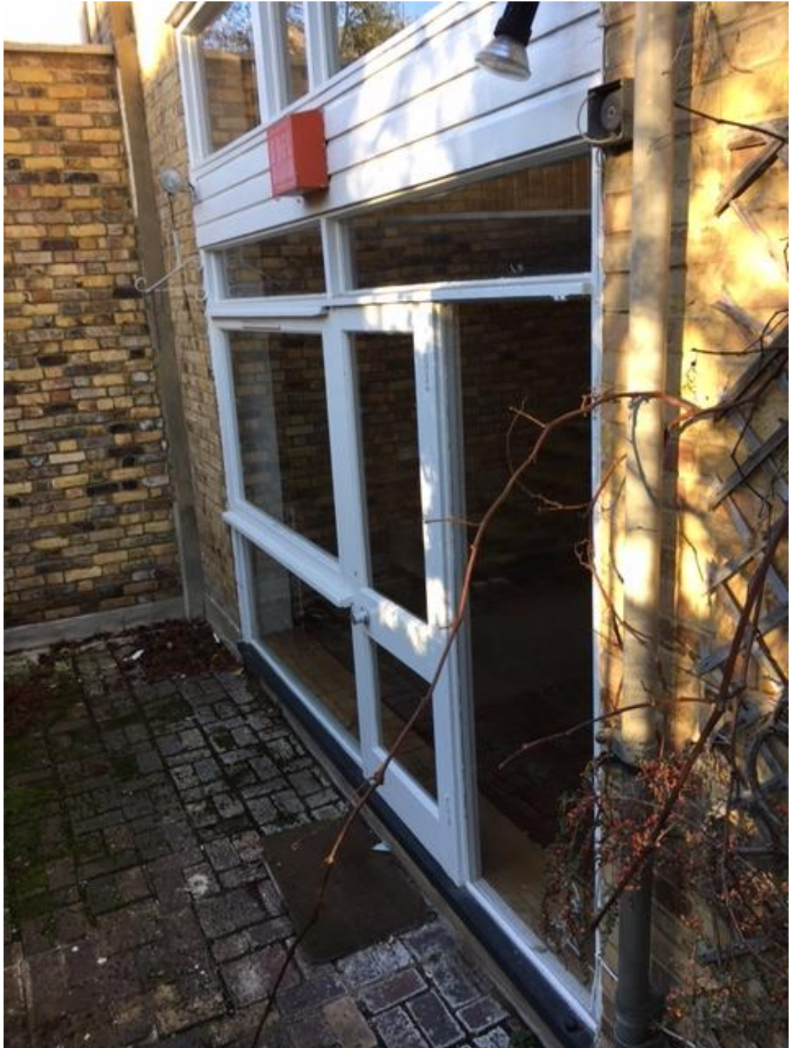
Photo 3- Existing Rear Elevation at no. 65
