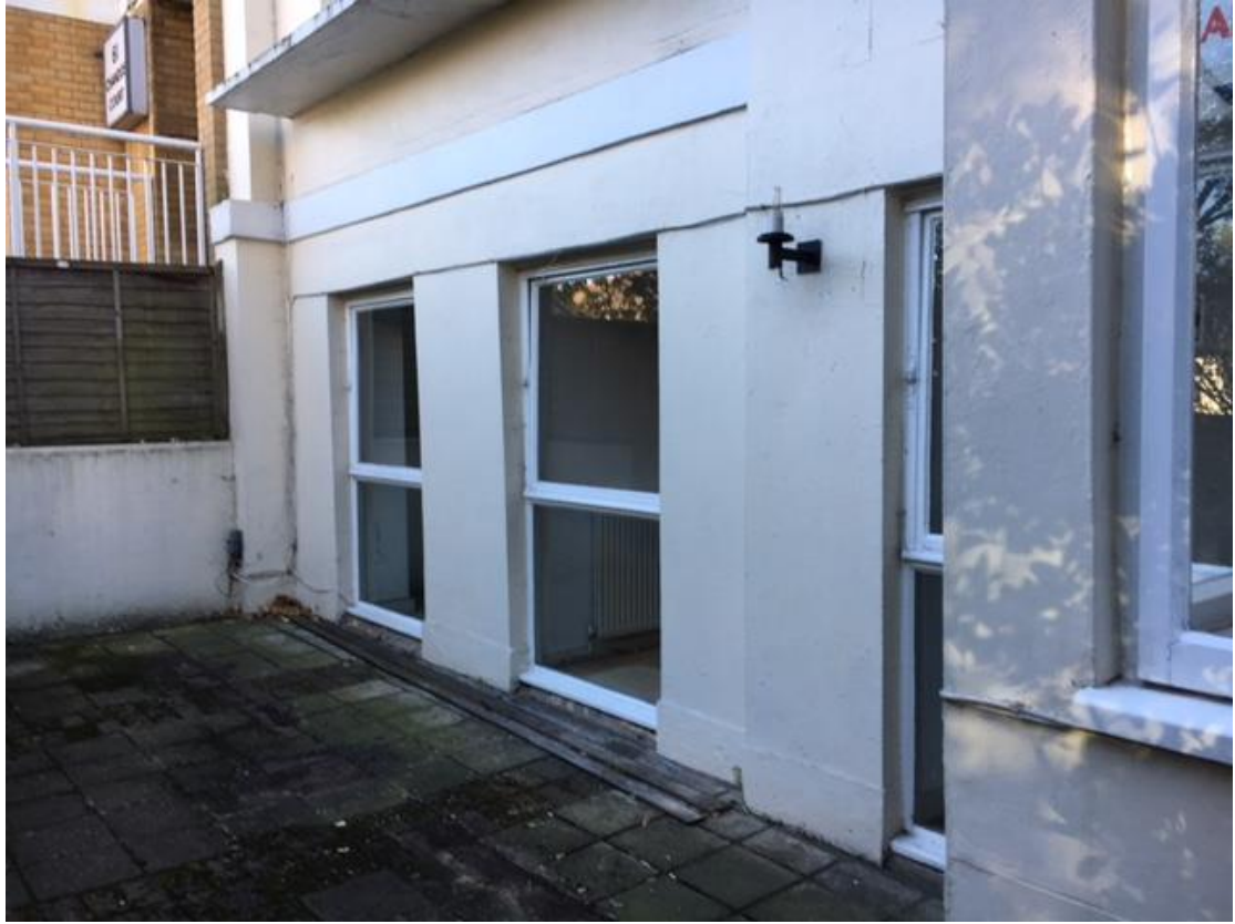
Photo 8- Existing Front Elevation of no. 63
