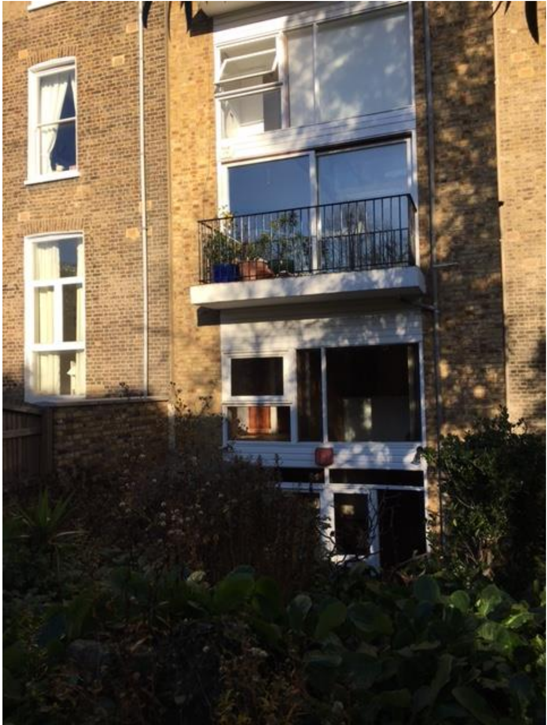
Photo 1- Existing Rear Elevation of no. 65
