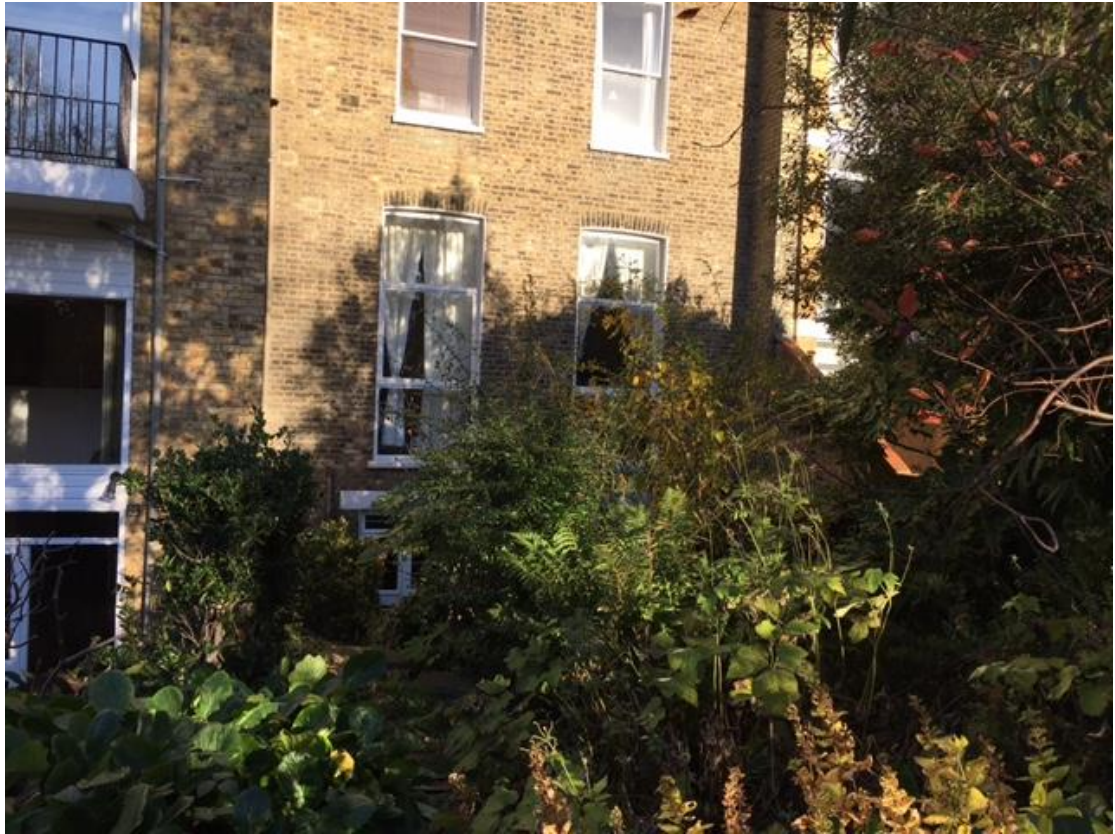
Photo 2- Existing Rear Elevation of no. 63
