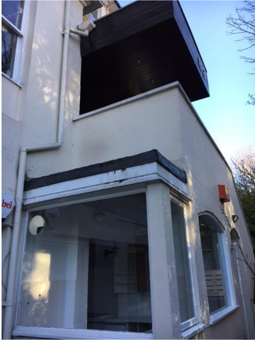
Photo 6- Existing Front Elevation projecting forward of the main front building line
