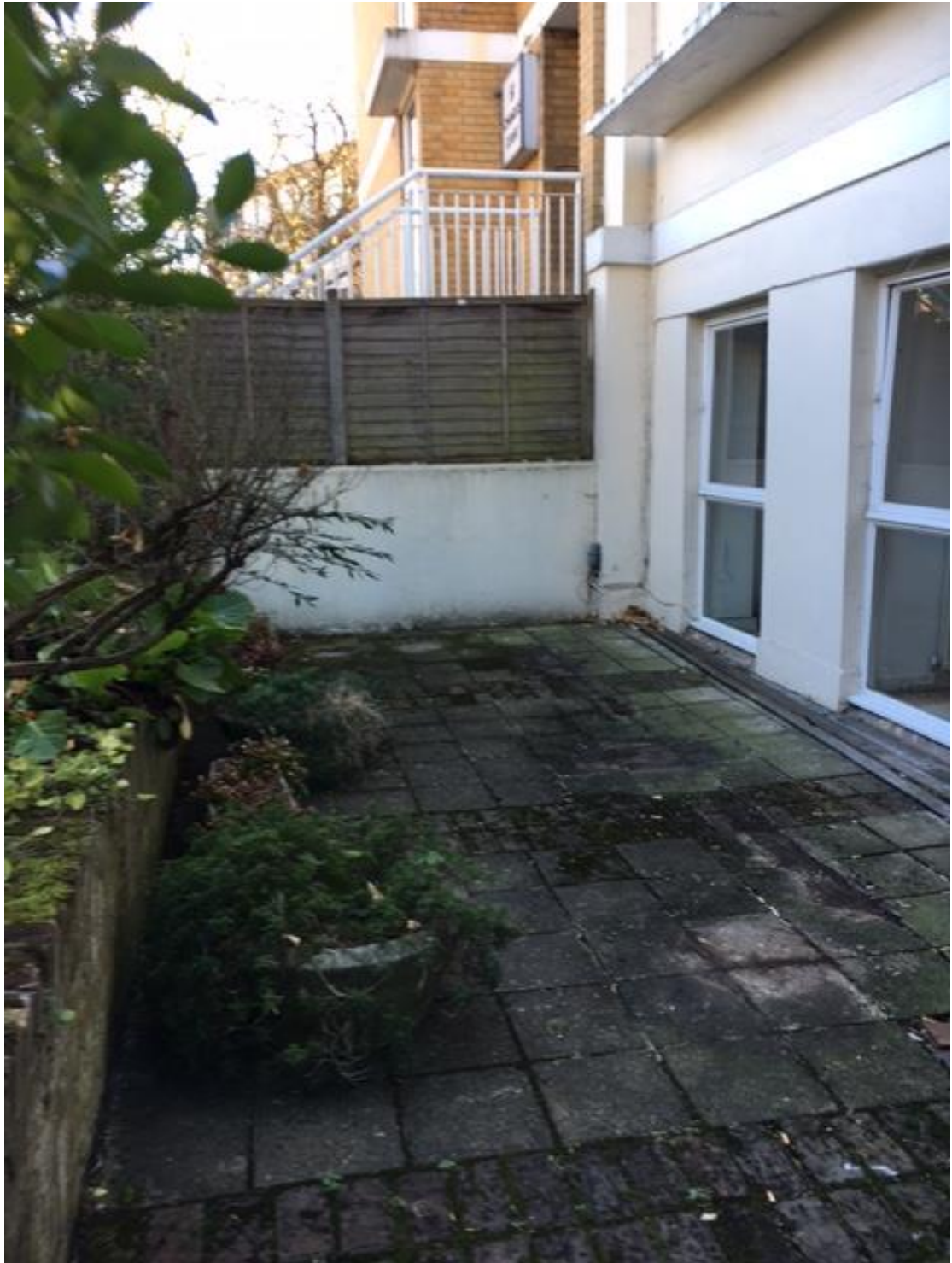
Photo 7- Existing Front Elevation of no. 63
