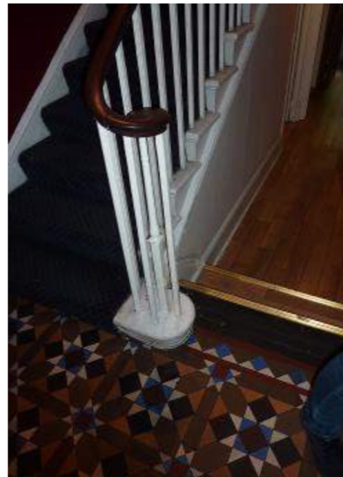
Figure 26: No. 77 Ground floor landing showing Victorian ceramic tile floor and plain geometric stair
