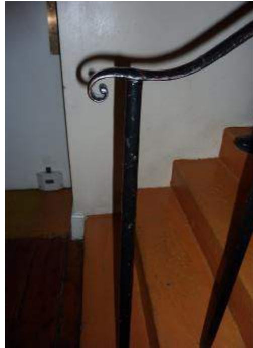
Figure 30: No. 79- the basement stair still retains its original wrought iron hand rail
