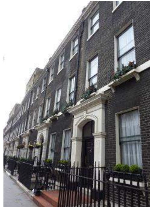
Figure 22: View South along Gower Street showing No. 79 to the right and 77 to the left
