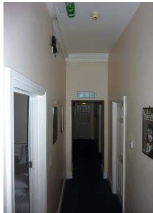
Figure 23: The plan form of the building has been severely eroded through the lateral conversion of both properties, much to the detriment of the understanding of the buildings' forms
