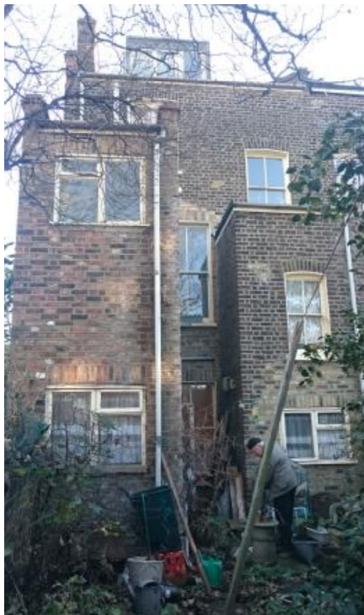
Photograph of existing building – rear elevation
