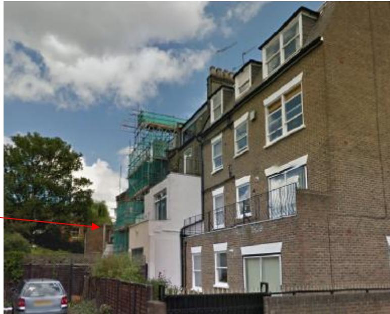
Rear of the subject terrace (Street View) including other rear extensions
