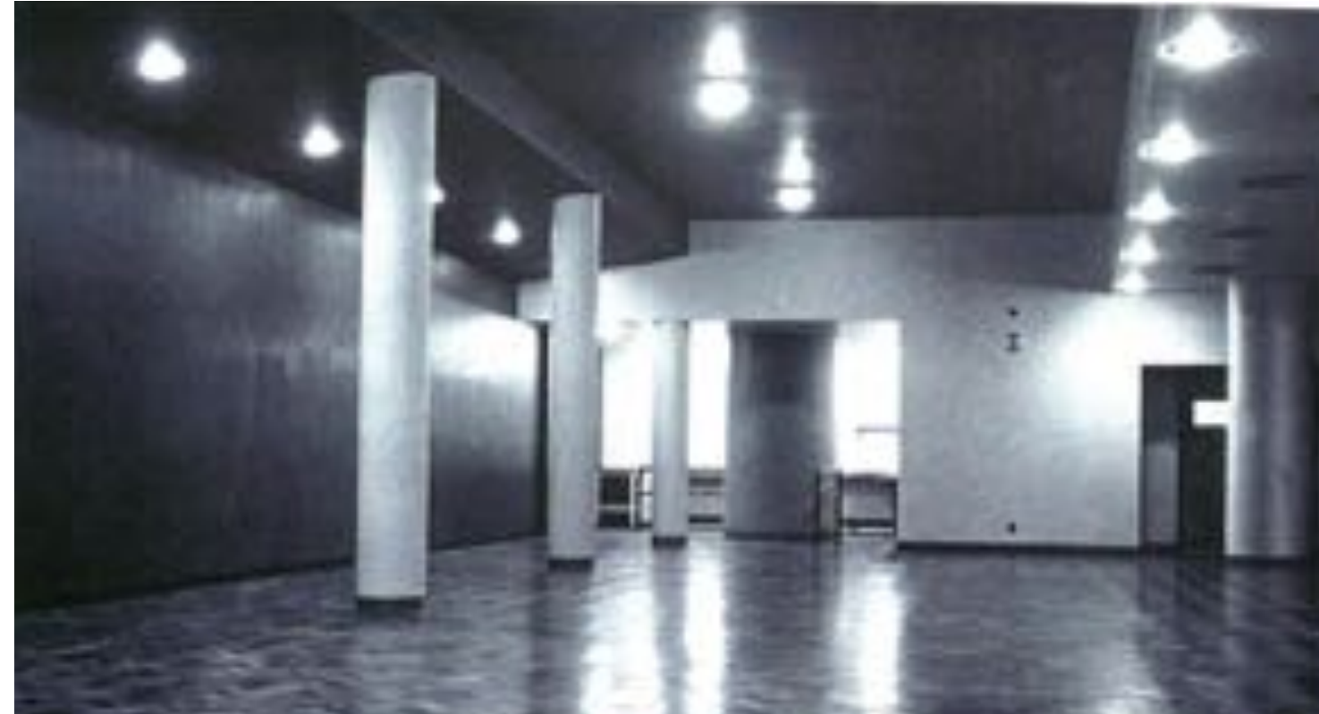
The canteen as designed by David du R aberdeen in 1958
