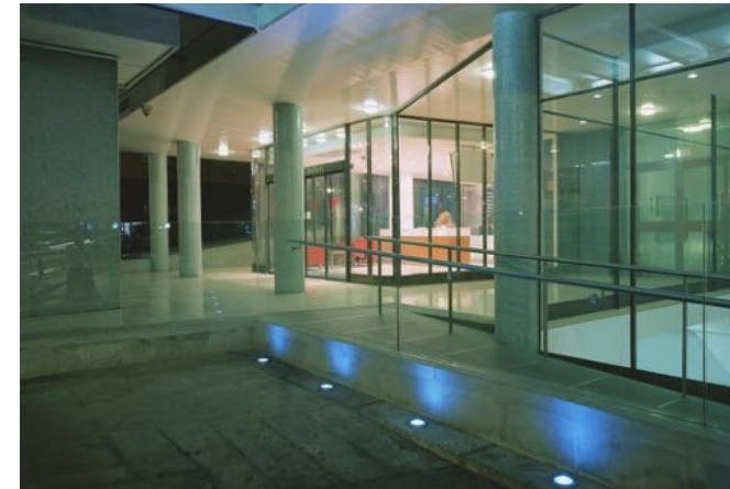
Disabled entrance ramp, installed 2004
