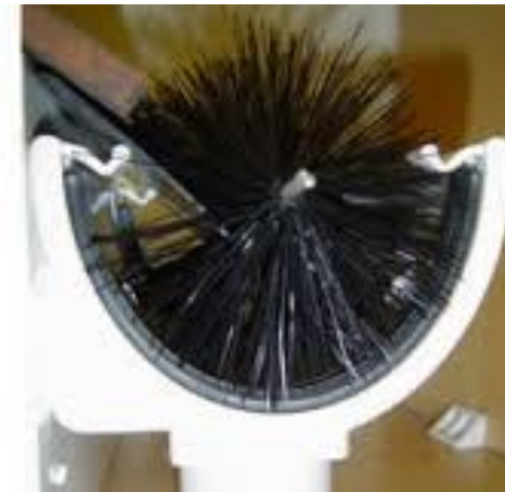
Fig 4 - Suitable gutter guards (2 types shown above) should be fitted to ensure that leaf drop from adjacent trees does not block new guttering leading to potential pressure for tree works.
