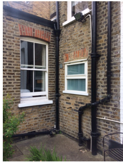
PHOTOS OF EXISTING WINDOW
