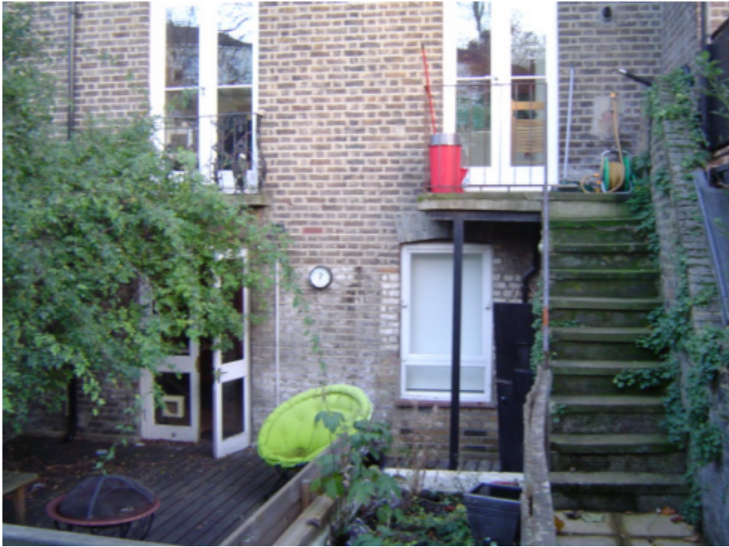
Rear of application building
