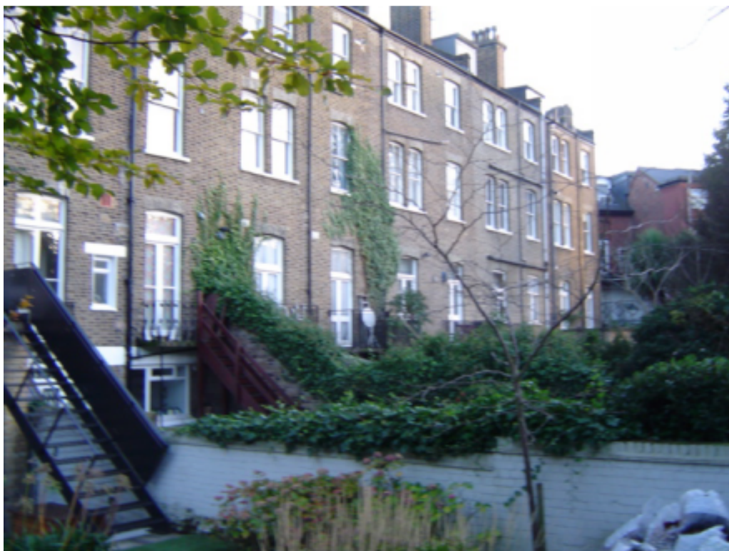
Rear elevations of the terrace
