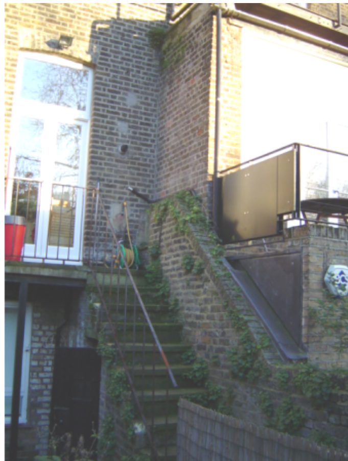
Existing staircase adjacent to the boundary with no.8
