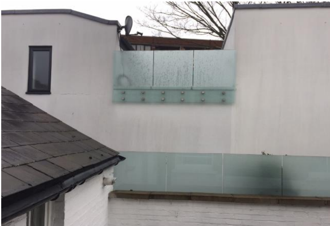
Beaumont Mews to the Rear of Charlton King's Road
