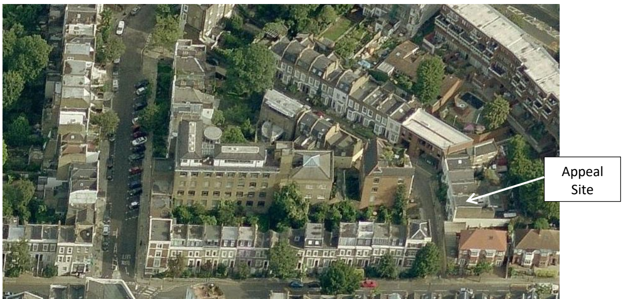
Aerial View of the Appeal Site and Surrounding Location
