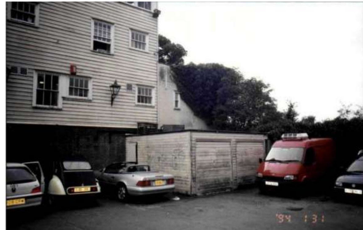
Figure 16 Garages to north-west corner of Jack Straw's Castle
