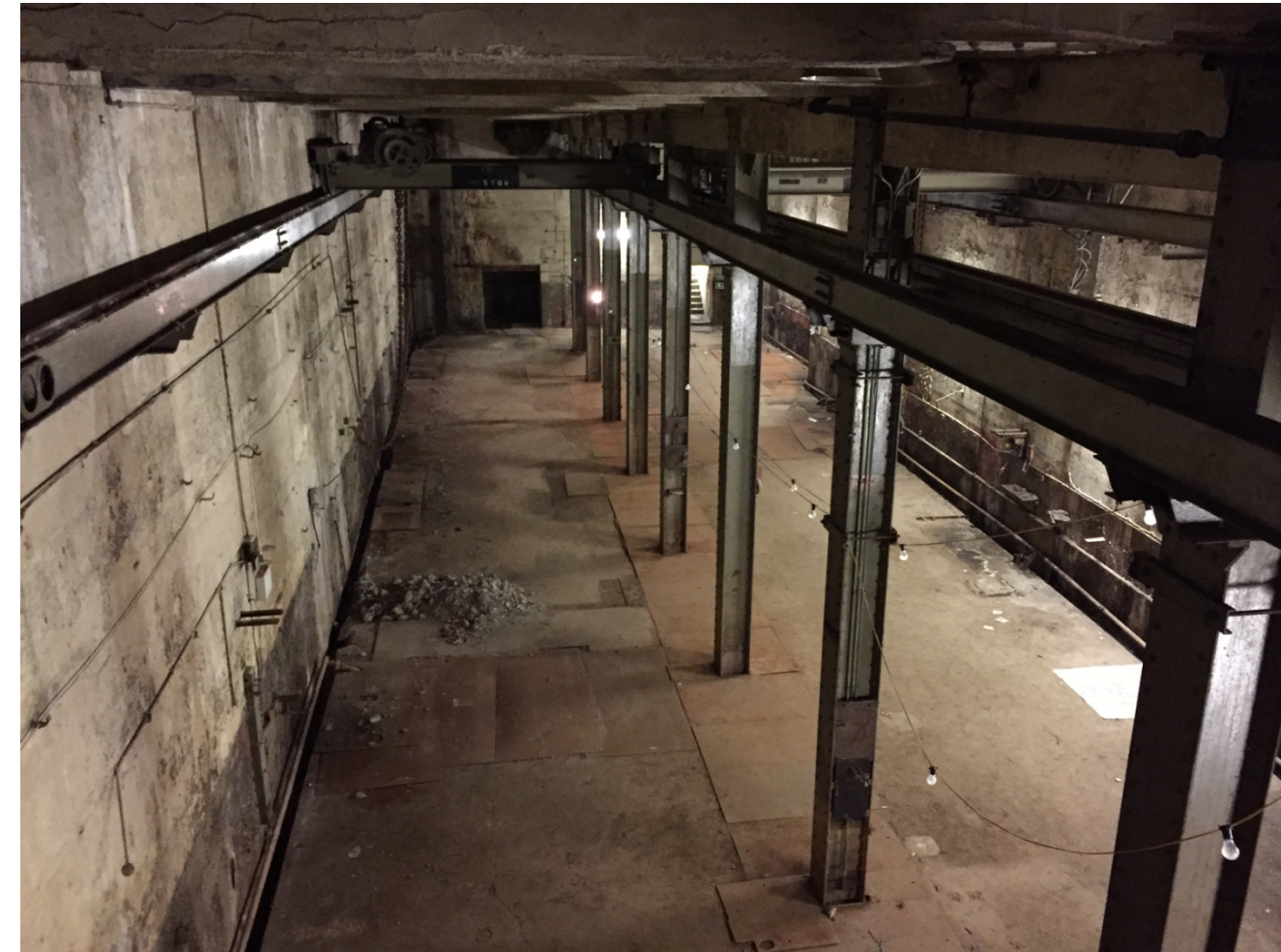
16.1 VIEW INSIDE EXISTING BASEMENT TAKEN FROM STAIRS
