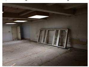
• Internal Walls: All existing walls and mouldings to be retained and redecorate with white paint; all exposed brick work walls to be covered with plasterboard decorated with white paint
