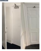
• External Front door: External door to building frontage to be retained and redecorated with white paint internally. Ironmongery retained. New access controls mounted to wall externally beside door.
