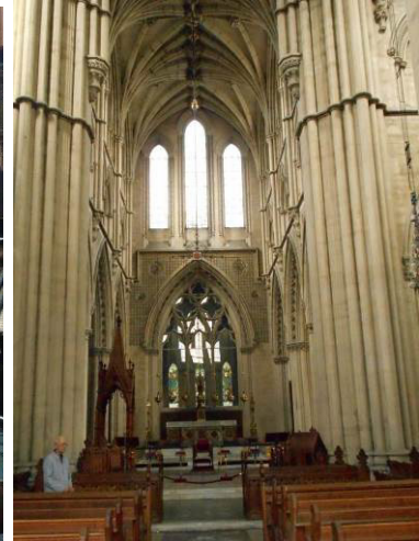
Nave looking East
