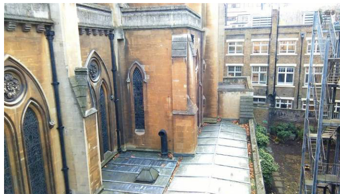
Existing boiler flue on rear elevation
