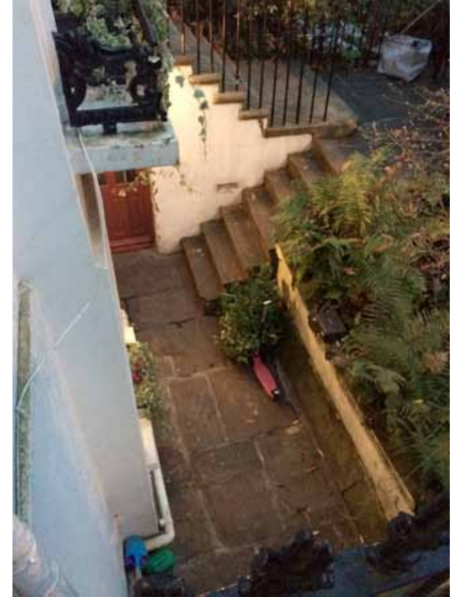
View of the adjacent house garden, showing the lowered area enlarged.
