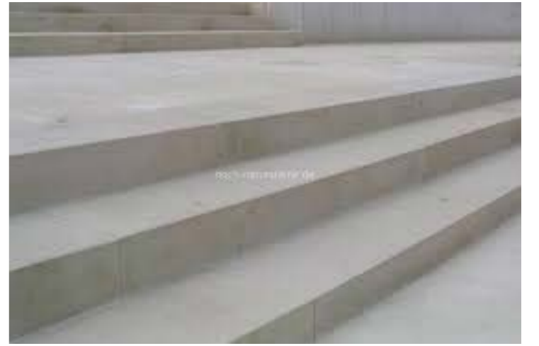
stone treads and risers
