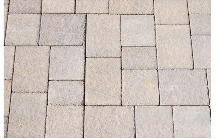
permeable interlocking paving
