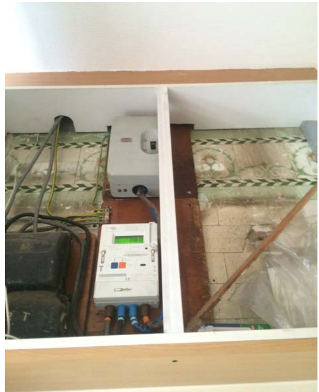
Tiles visible within meter cupboard
