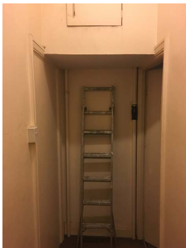
Large service boxing at no. 45 - to be removed.
