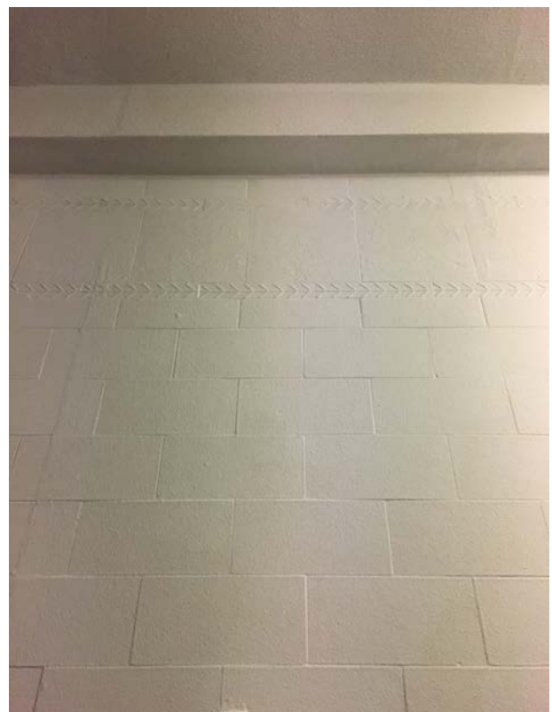
Outline of tiles can be seen beneath paint
