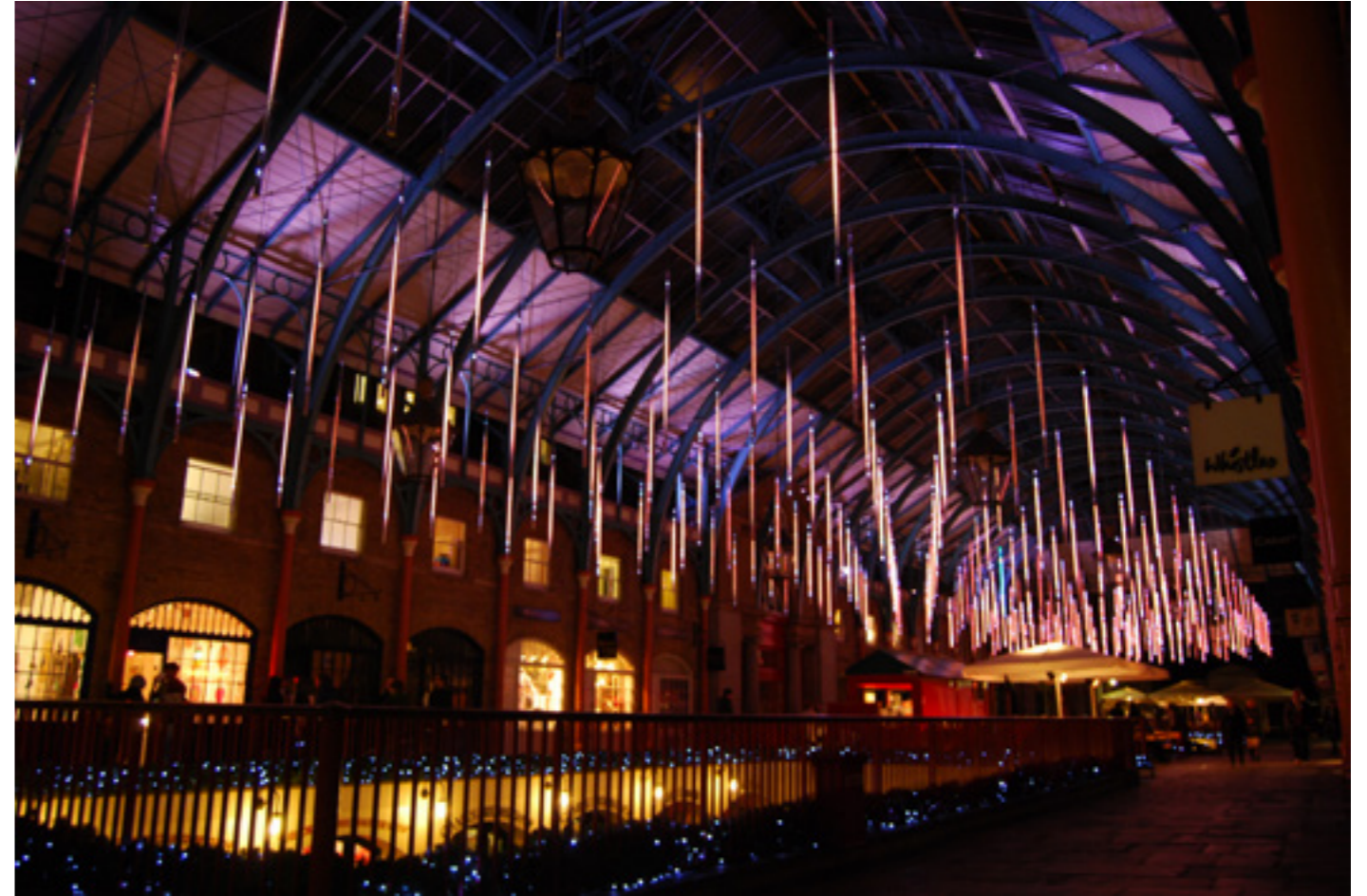
Reference image of specially commissioned seasonal lighting installation
