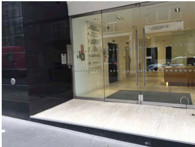
Photograph 2 - Entrance to Baird House foyer via manual & push-button operated swing doors
