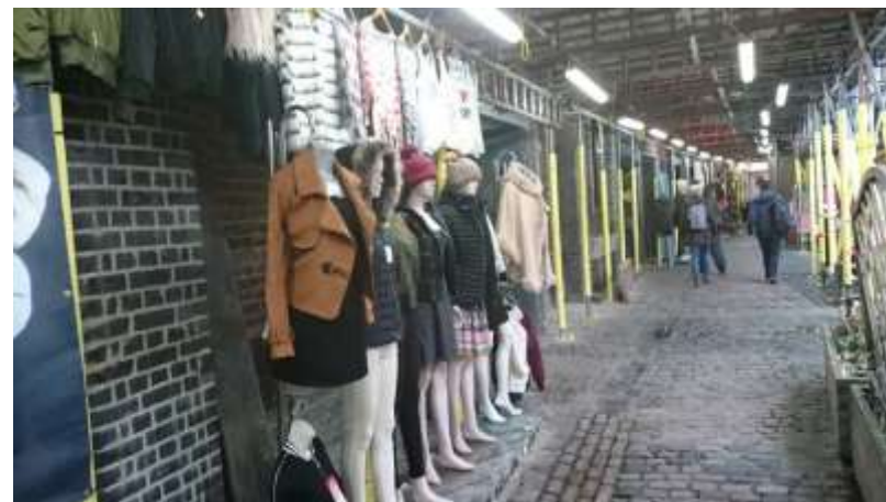
Figure 6: Chalk Farm Building facing east, units 29-35 on the left (January 2017).
