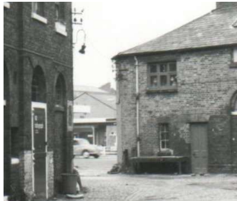
Figure 4: 1975 photograph looking north towards the former gatehouse end of the Chalk Farm building.
