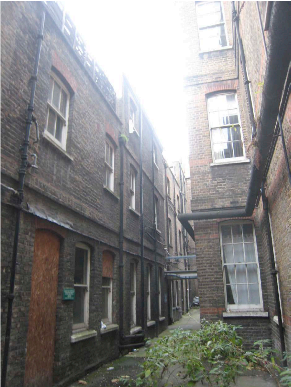
The South Wing: looking towards front
