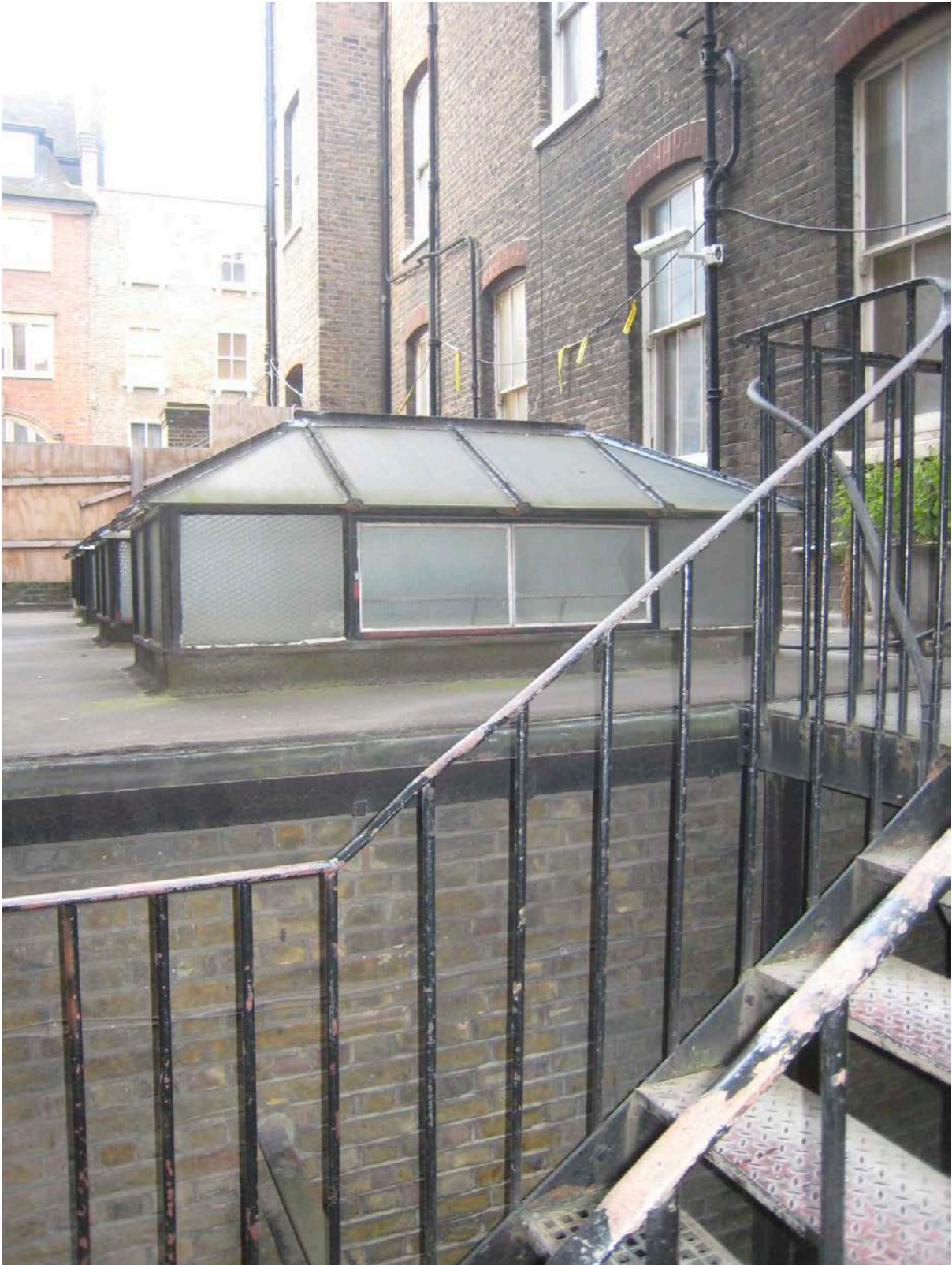
The North Wing: lower ground floor extension
