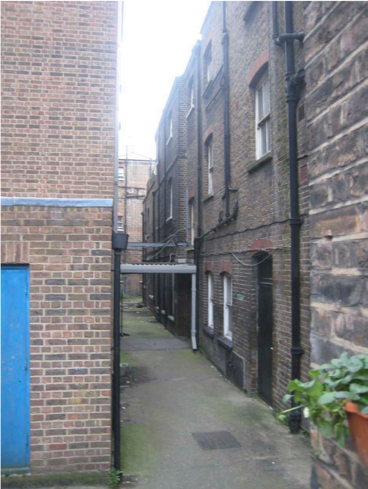
The South Wing: looking towards rear
