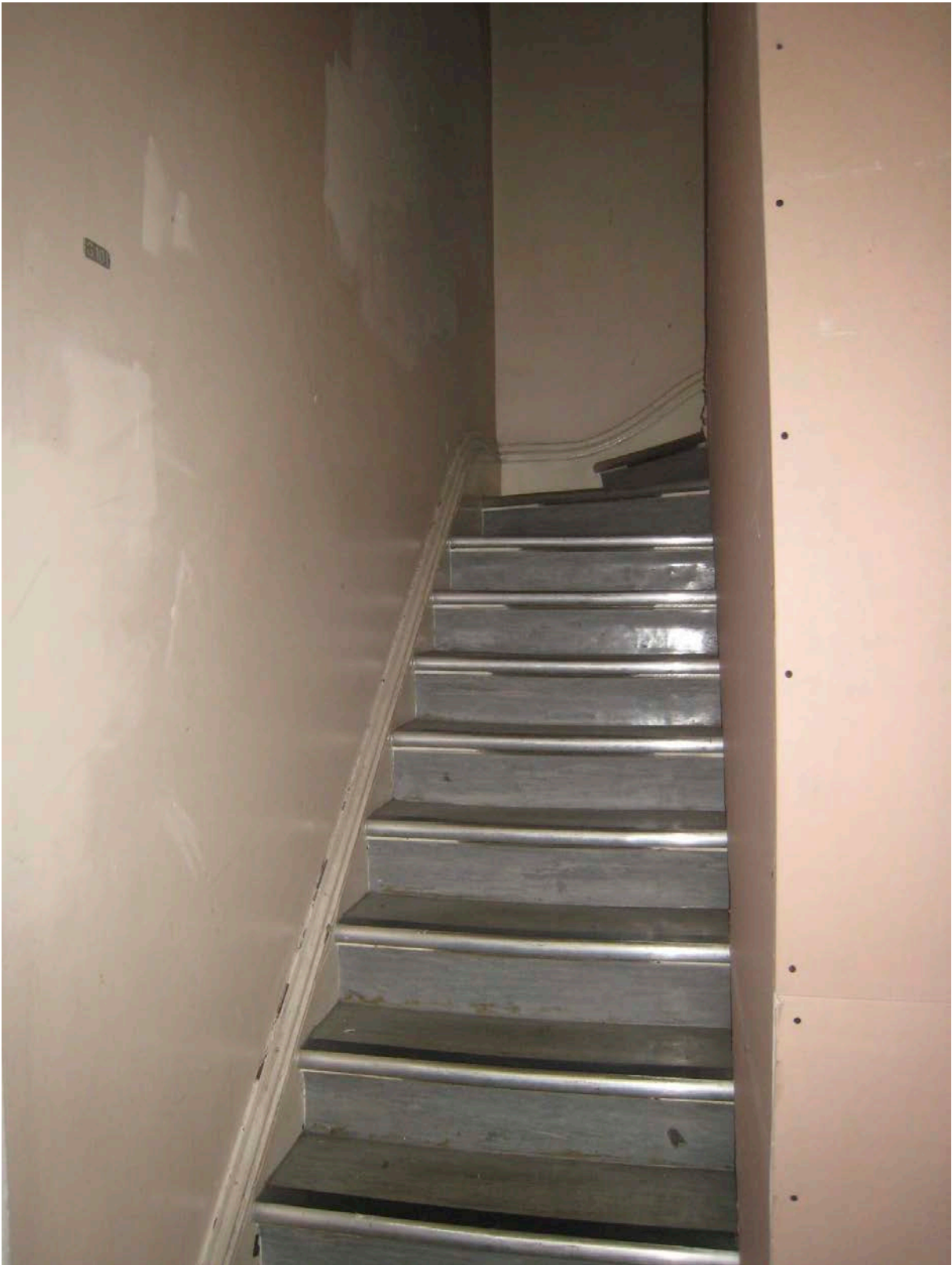
The South Wing: interior
