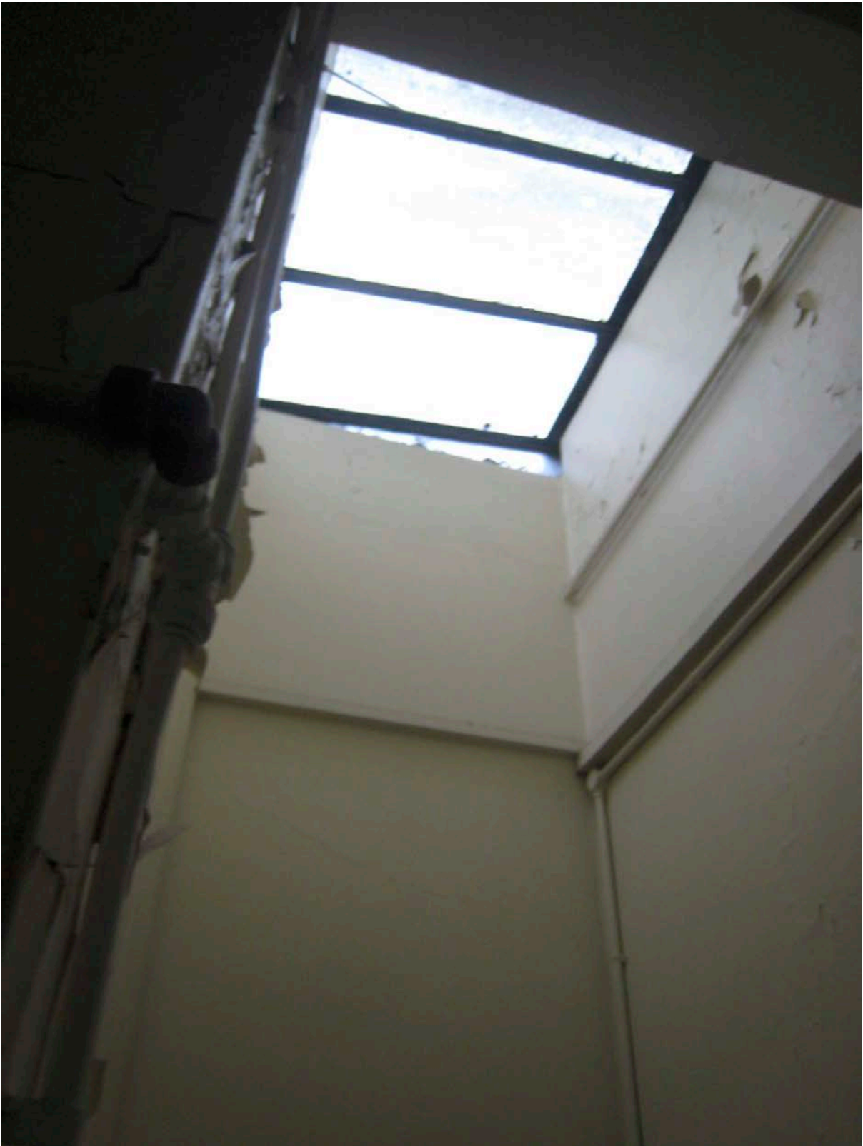
The South Wing: interior
