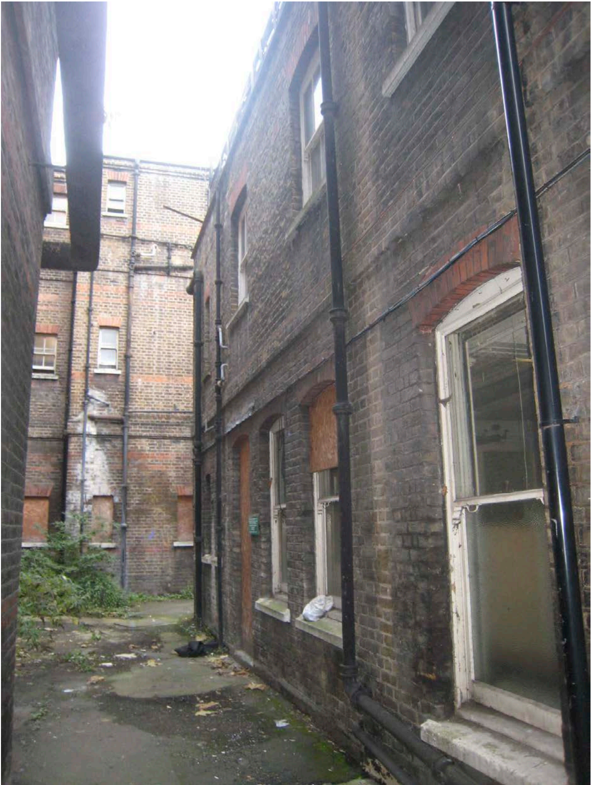
The South Wing: rear part
