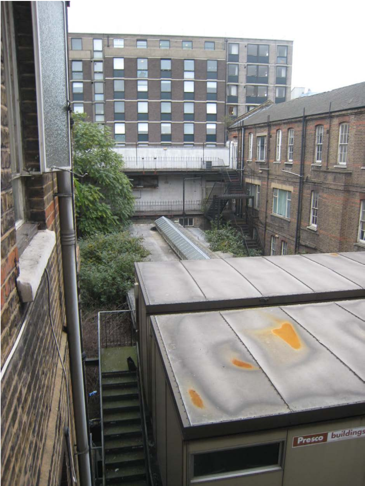
The east 'courtyard'
