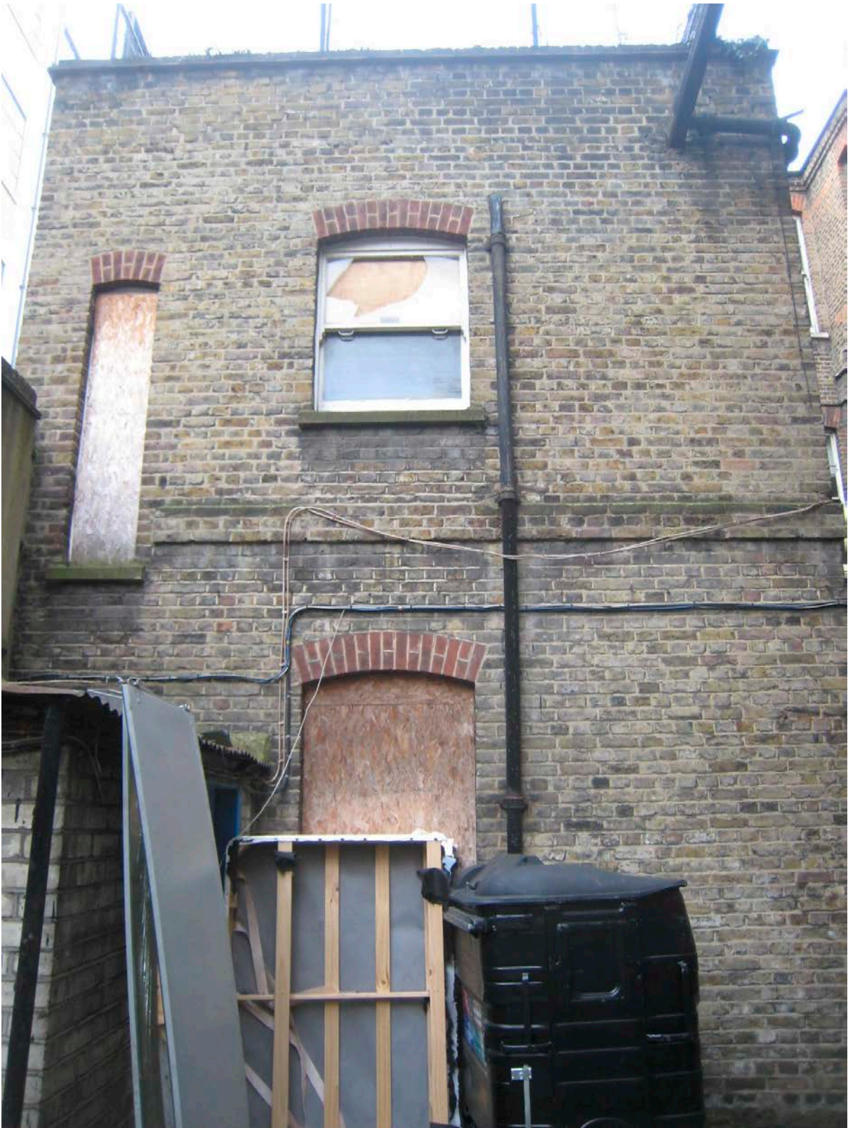
The South Wing: rear part
