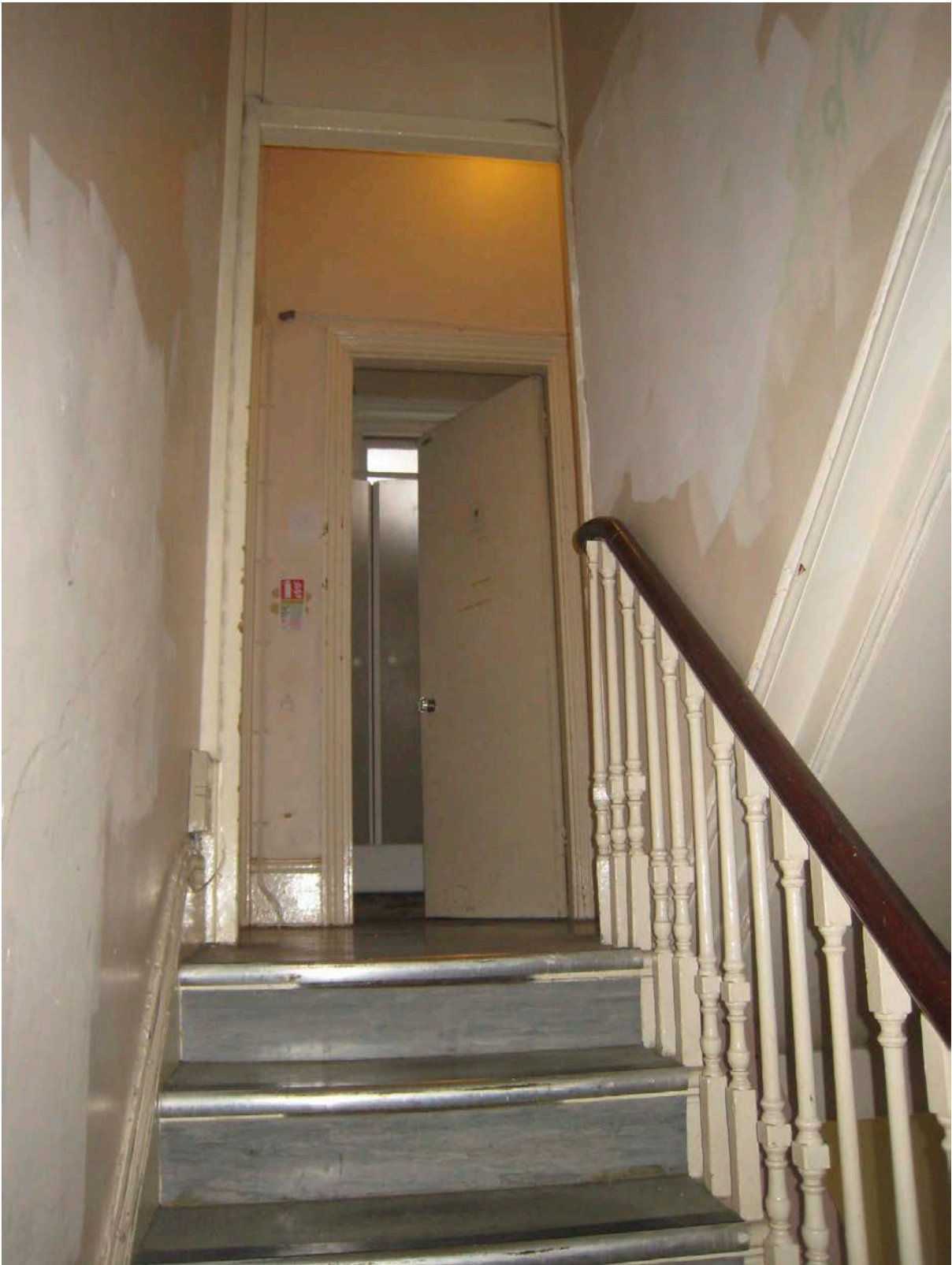
The South Wing: interior
