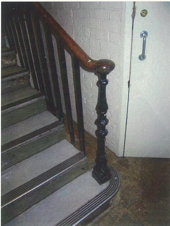
Fig 26 Cast iron newel to south stair
