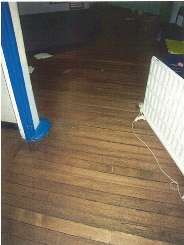
Fig 28 Interior ground floor 1880s? north wing – floor boards. One of the few places where original finishes are visible.
