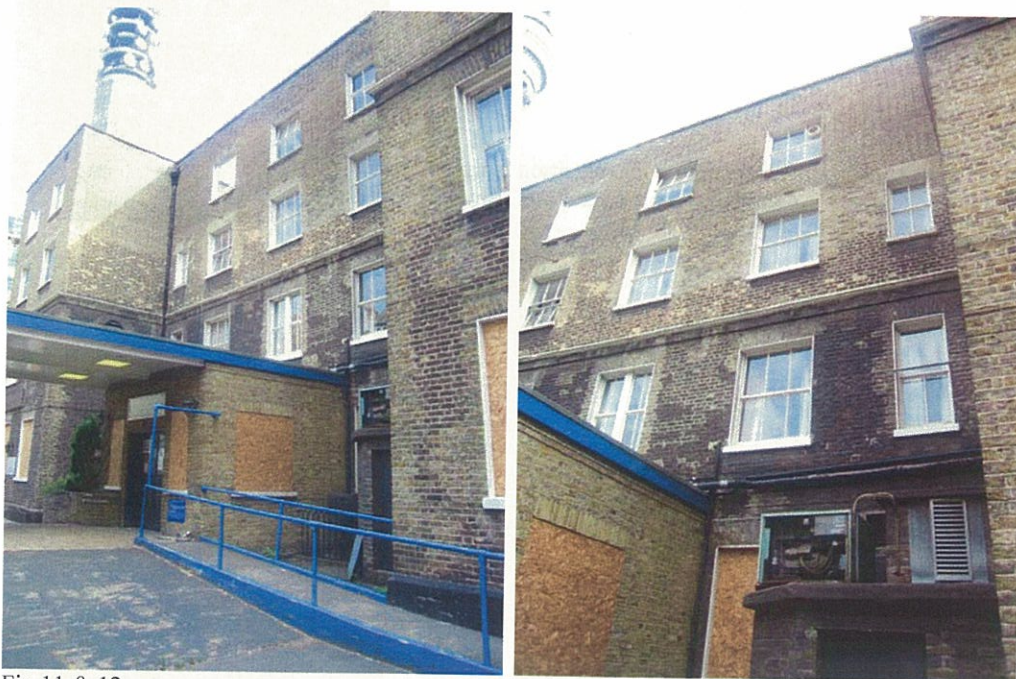
Fig 11 & 12 General view of main entrance with 1950s? porte cochère. Note different brickwork above string course and second floor bottom hung window sashes.
