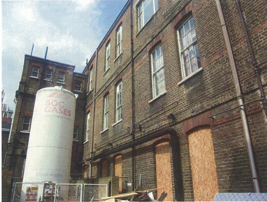
Fig 19 South wing, south elevation, with red brick bands and rubbed red brick window arches, toilet block to left
