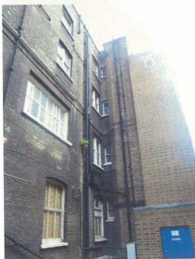
Fig 15 Original South front with Portland stone string course transformed into Platt band and with some original window openings. Beyond lie the 1880s extension and twentieth century lift shaft to right
