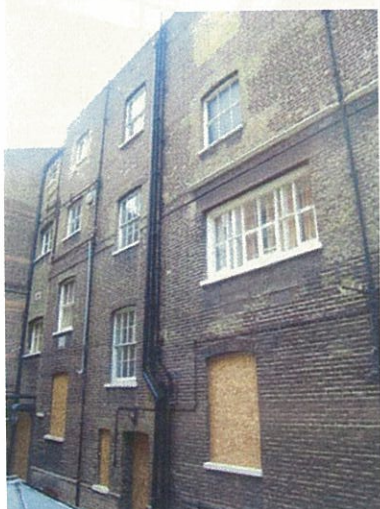
Fig 14 Original north elevation with main front second floor cornice returned into platt band
