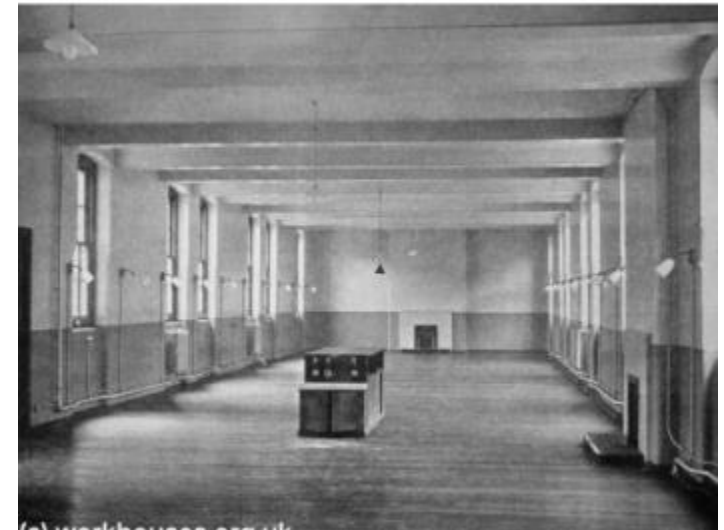
Refurbished pavilion ward of Middlesex Hospital Annexe in 1926
