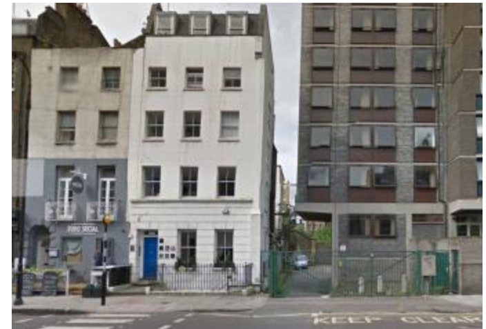
'Bedford Passage' from Charlotte Street
