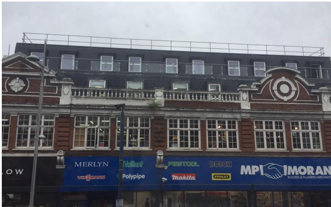
Figure 2 Recently completed roof extension at 293-301 Kilburn High Road opposite the site
