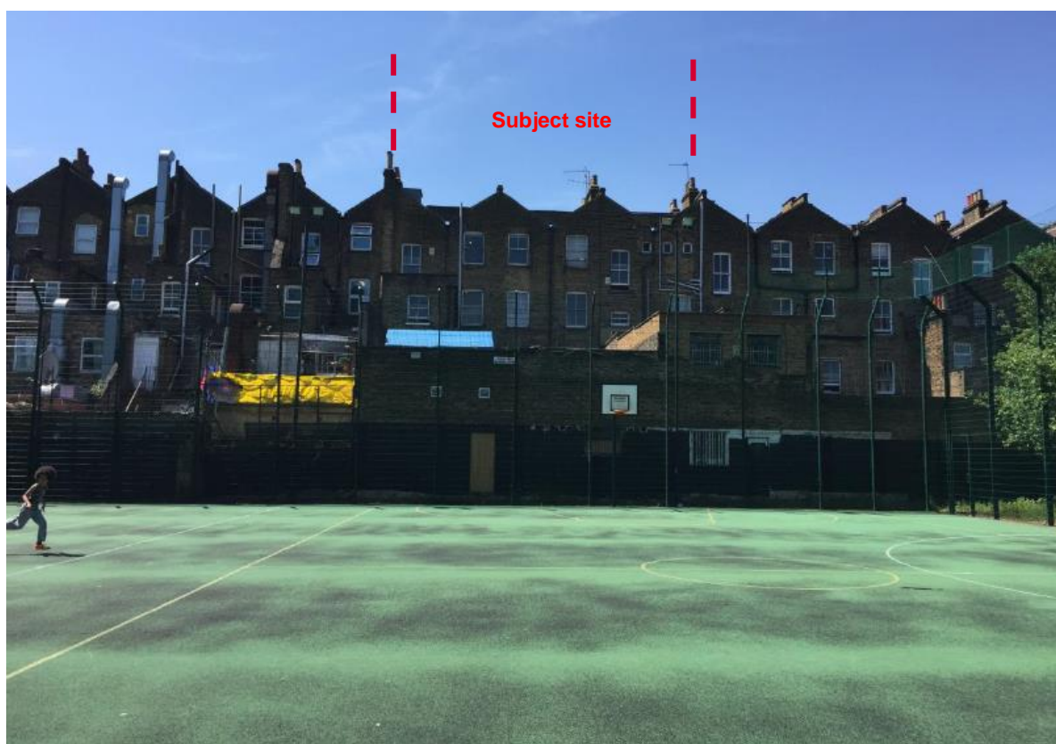
Figure 1 Varied nature to the rear of the terrace
