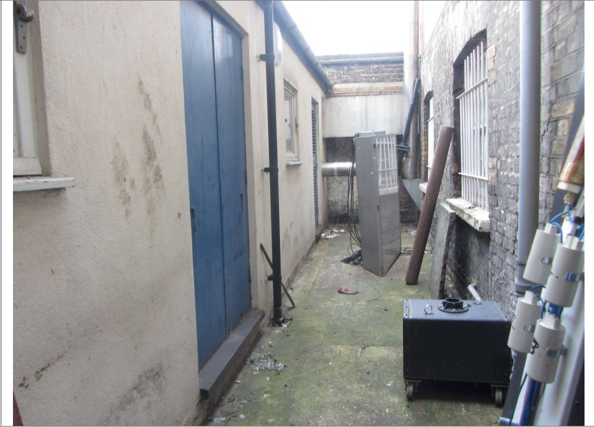
Photo 5: Rear hardstanding yard at lower ground floor level
