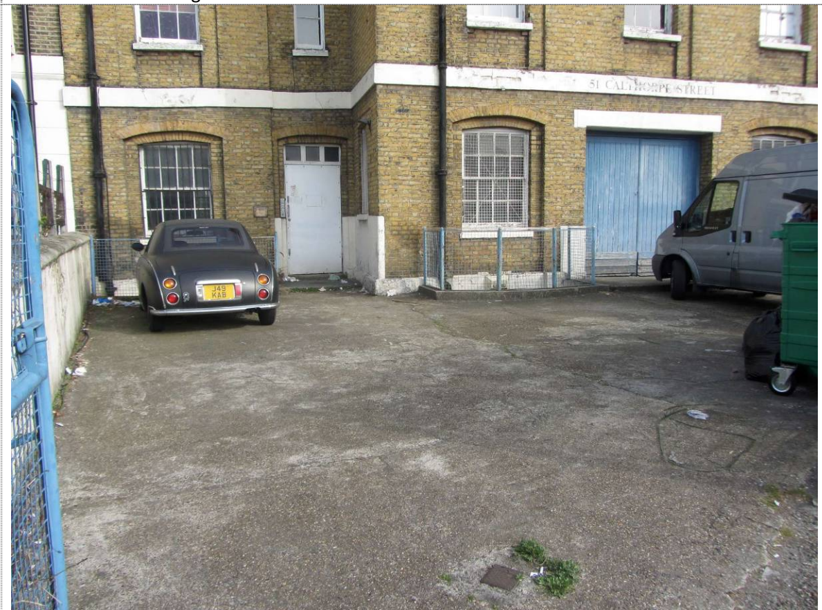
Photo 2: Front hardstanding courtyard & boundary with No.49
