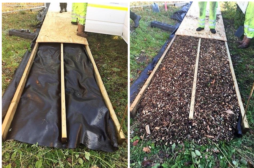
Figure 4. Plywood sheeting used as ground protection.
