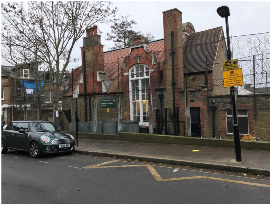
Pic. 2 – Dornfell St (north-east)- school's building which is used as their commercial kitchen
