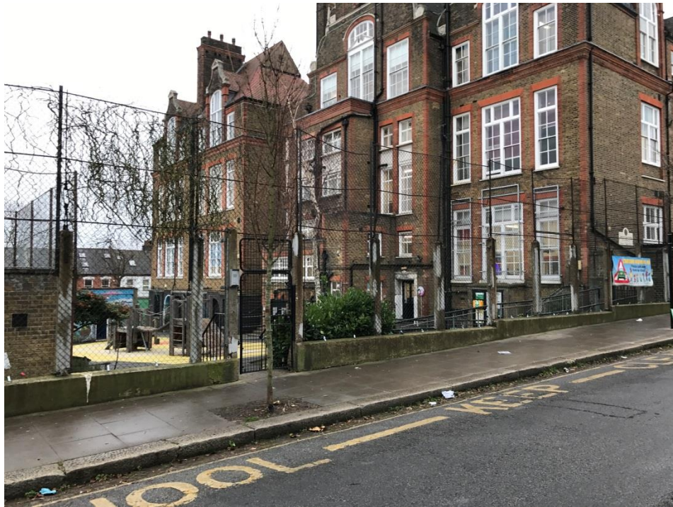
Pic. 3 – Dornfell St - school's existing chain-link fencing with pedestrian gate
