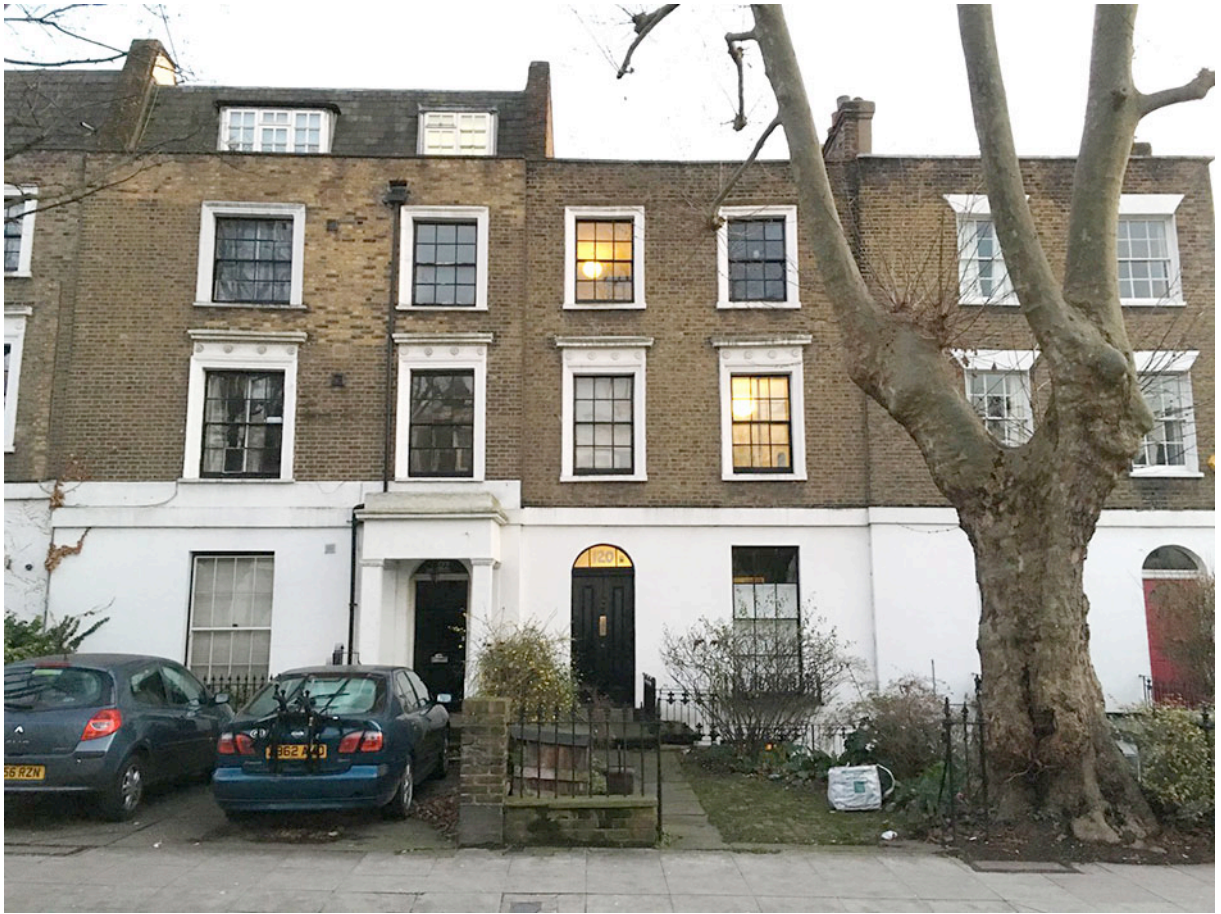
Fig.1 View from Leighton Road - front elevation of the houses No. 122, 120 & 118
