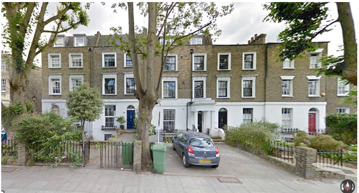
Fig.2 View from Leighton Road - front elevation of the terrace, houses No.126, 124, 122, 120 & 118
