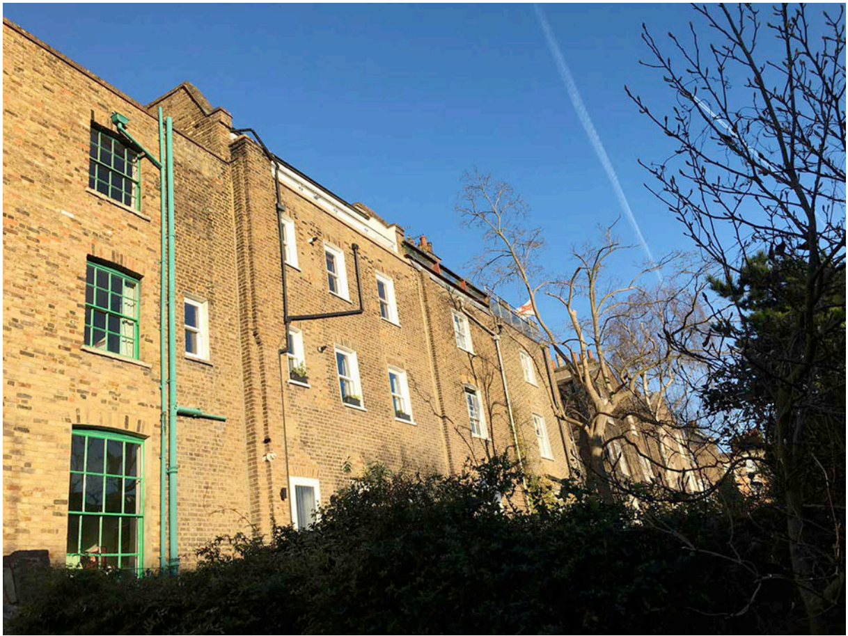
Fig.3 View towards rear elevation of the houses Leighton Rd No.120, 122, 124 & 126
