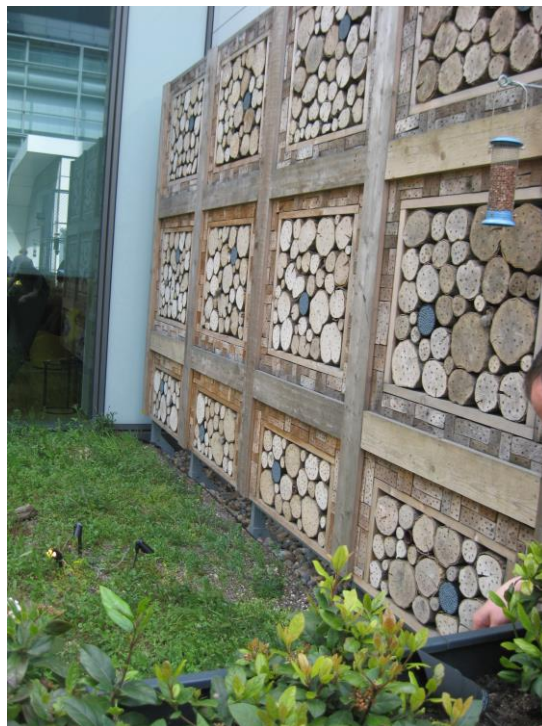
Photograph 5 Example of an invertebrate wall. (Photograph source: Rosie Whicheloe The Ecology Consultancy)
