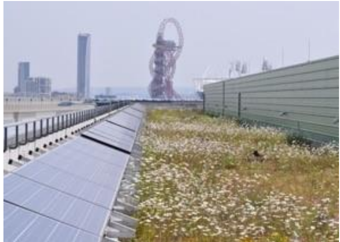
Photograph 4 Example of a biosolar roof. (Image provided by Dusty Gedge The Green Roof Consultancy).
