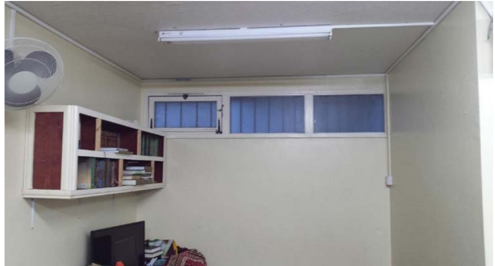
Photo 4 (above) : Ground floor room interior
