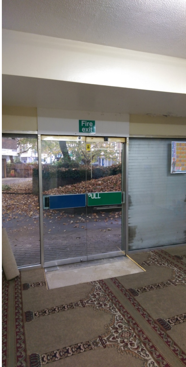
Photo 8 (above): Ground floor fire exit
