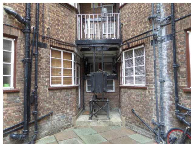
Typical Hoist, now redundant.
