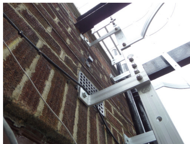
Example of renewed fixings to balcony
