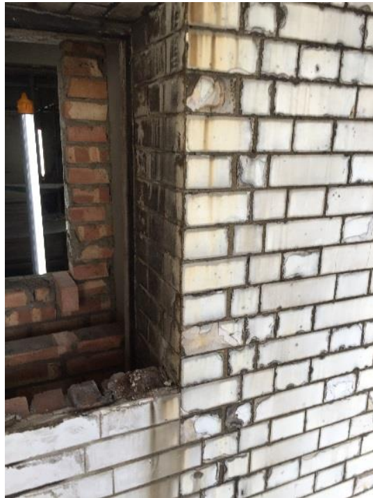
After removal of ductwork
