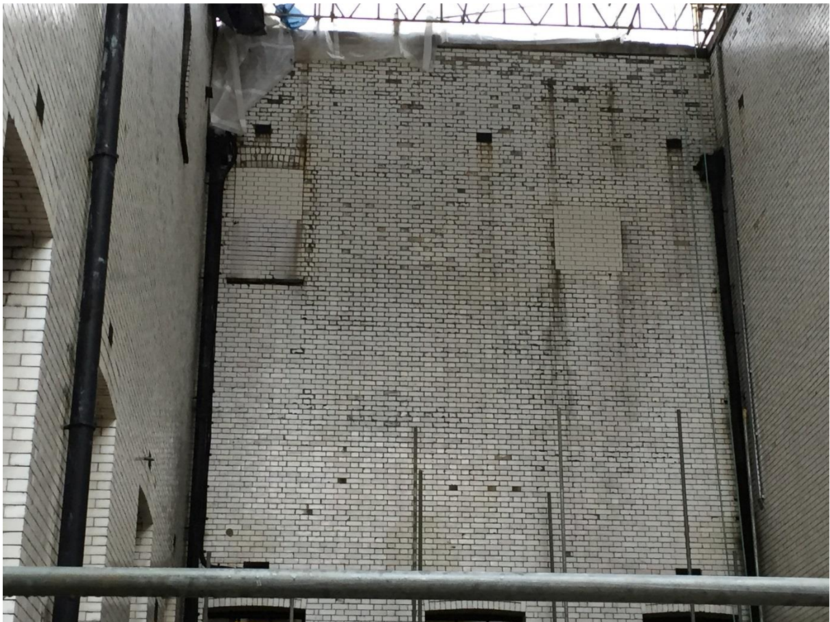
The completed glazed brick works
