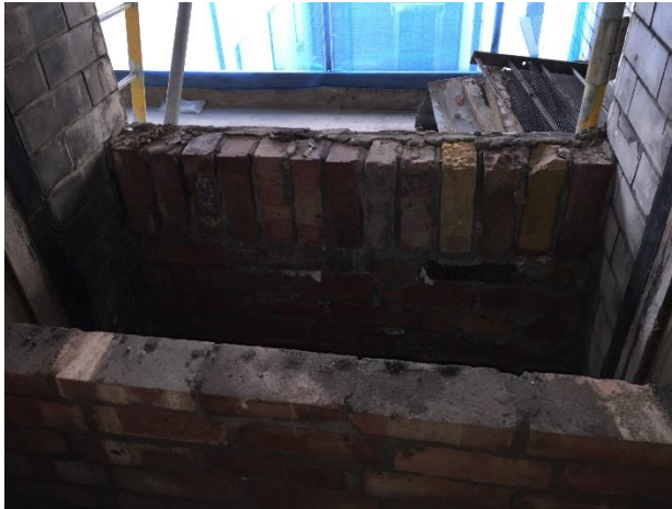
View from inside gallery after duct removed
