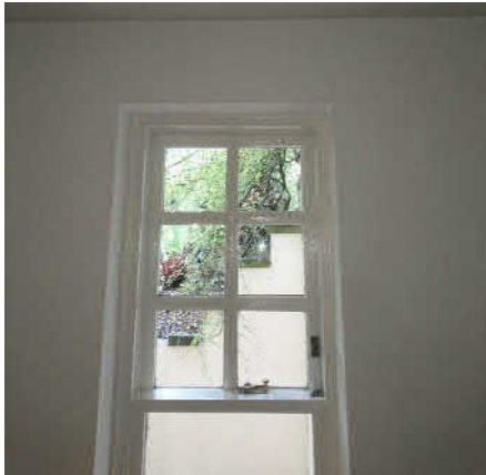
Photo 1 - Rear Wall Internal
