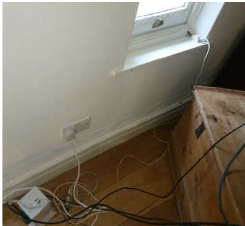
Photo 3 - Repairs to Waterproof Membrane
