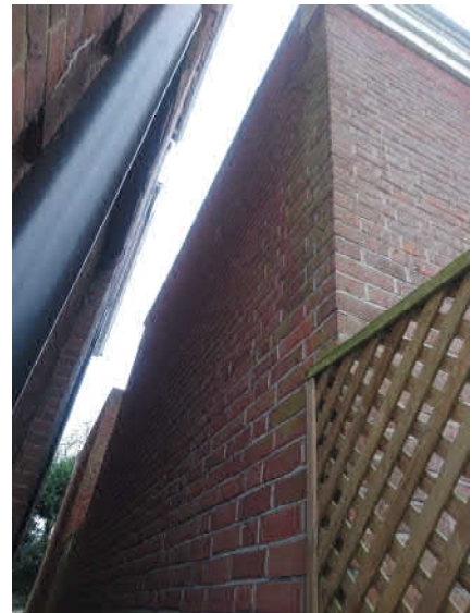
Photo 4 - Side Wall Property External
