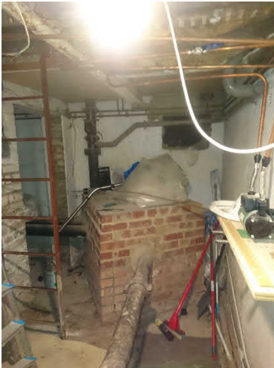
Photo 9 – Access to basement crawl space
