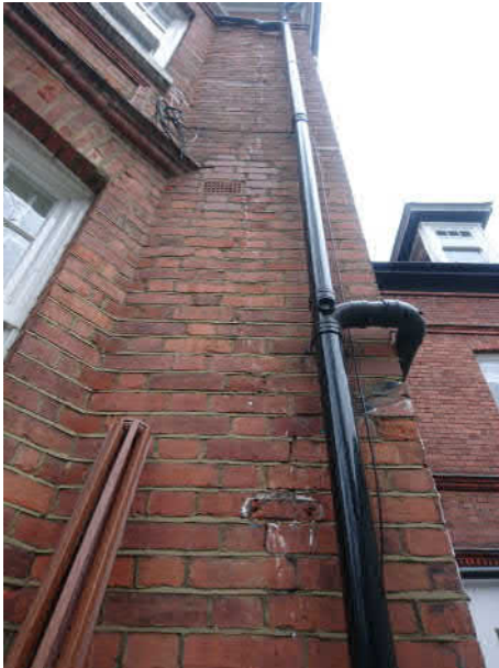
Photo 11 – Rear of property external
