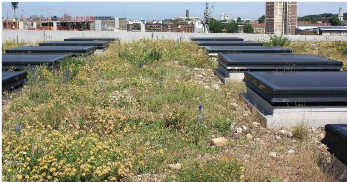
Figure 6: Simple brown roof system
