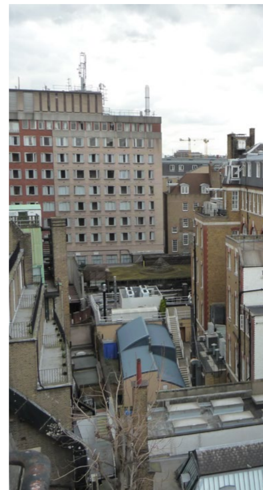
The view from the fire escape staircase on the back of the Hotel, looking north.
