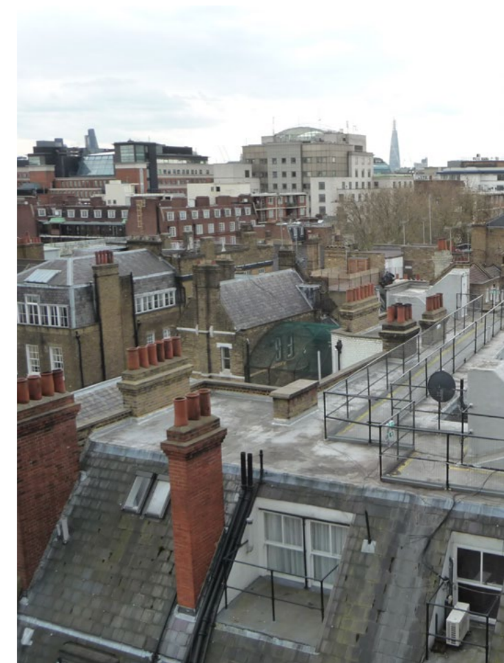
The view from the rear staircase, looking south.
