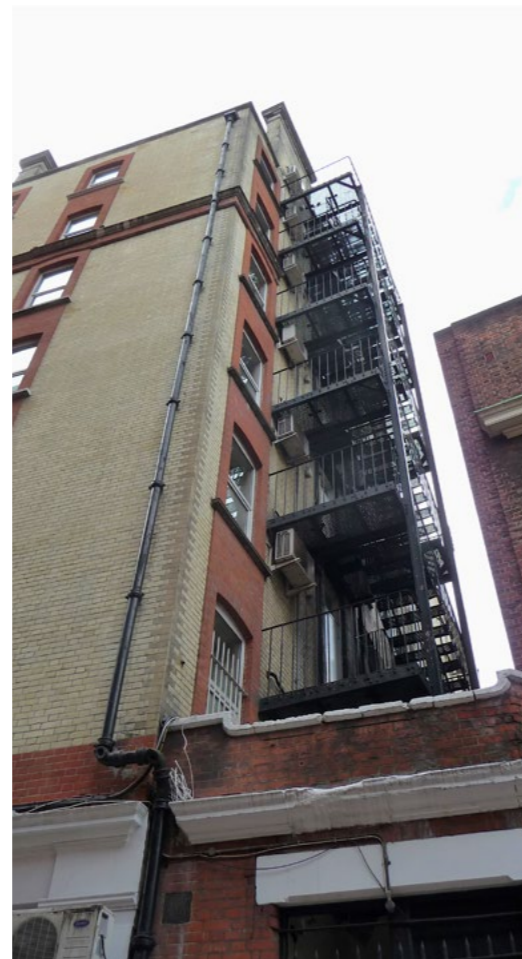
The fire escape staircase on the building's rear elevation.
