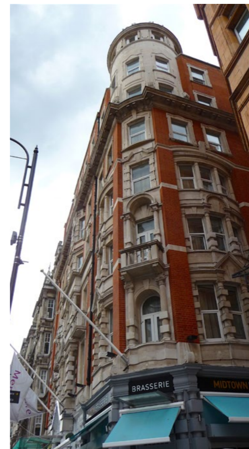
From close quarters, the roof extension would not be visible, as is already the case for the 7th floor.
