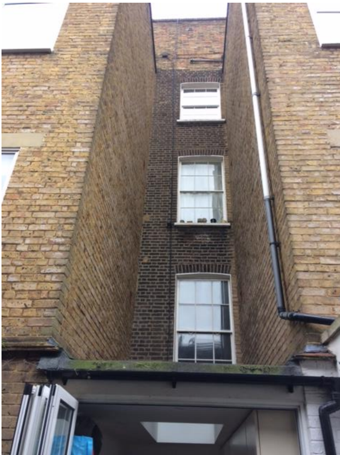
Photo 2: Rear elevation lightwell at first/second floor.
