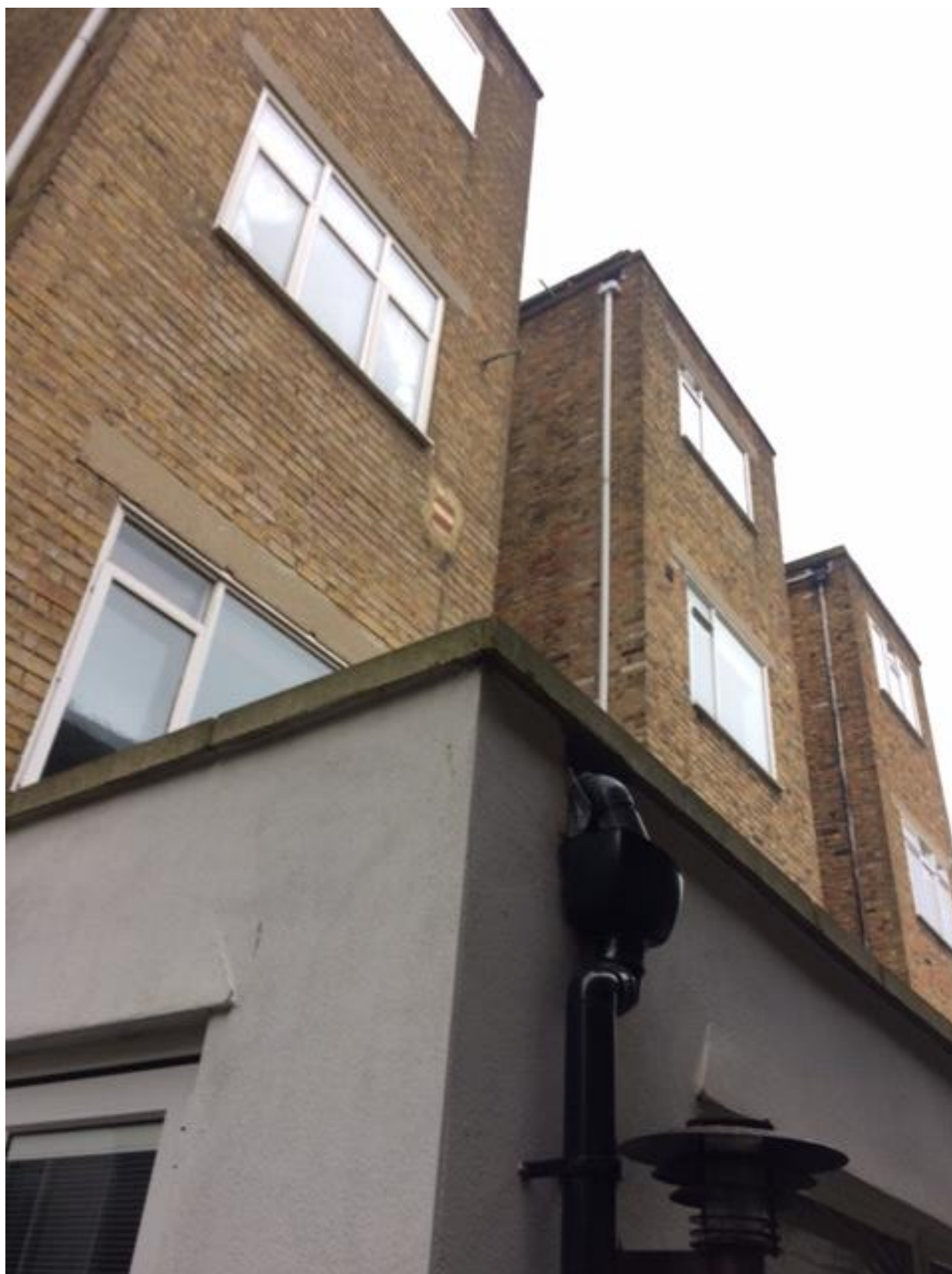
Photo 3: Rear elevation showing upper floors and neighbouring property to the north.
