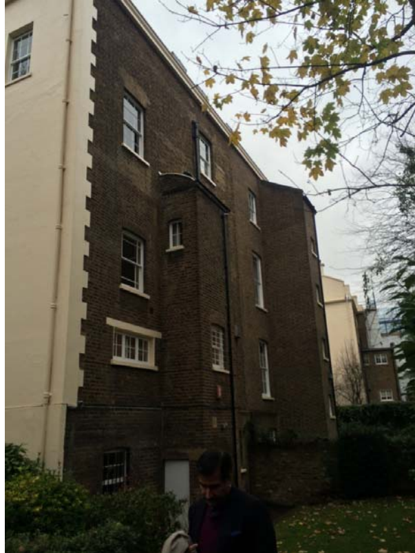
Existing rear facade
