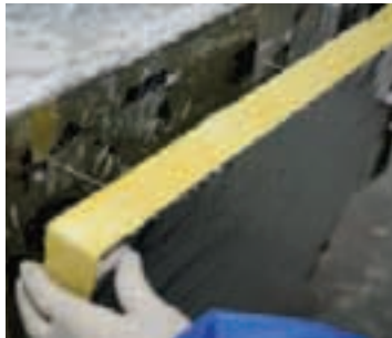
Isover CLIMCOVER slab installation
