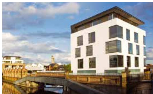
Westbourne Grove Canal Building, London
