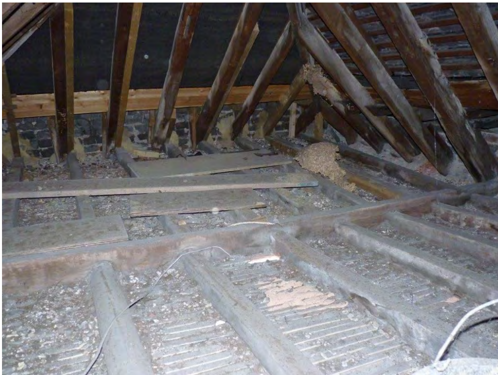
Ceiling showing original lath and plaster and ceiling joists
