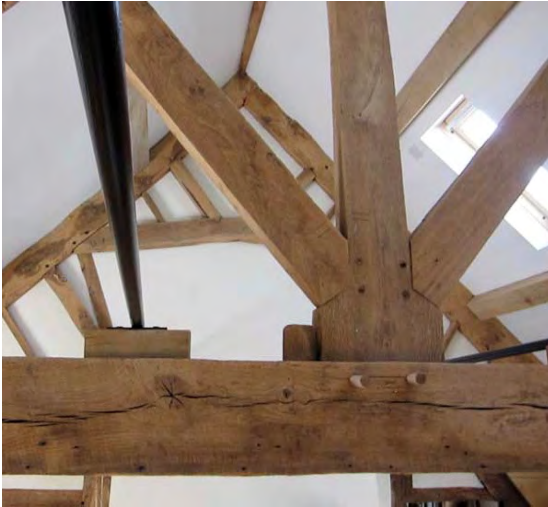
Example of ceiling removed in a timber-framed listed building (web image by Apex)
