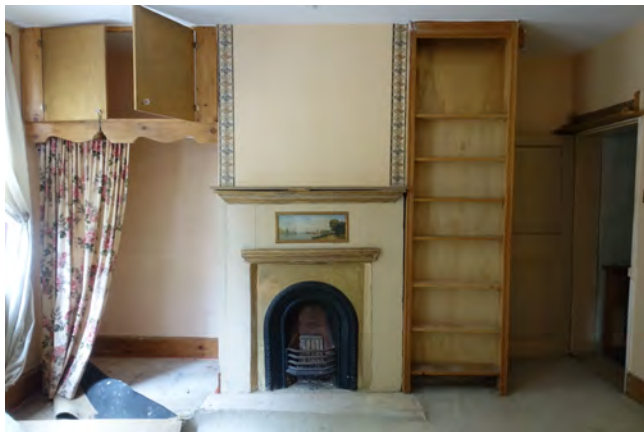
First floor bedroom Remnant of eighteenth century panelled fire surround with nineteenth century cast-iron inset. Modern cupboards on north wall. Salvaged/distressed timber mantels applied, modern marble hearth
