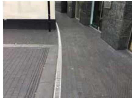
A - Change in ground surface outside existing A3 units
