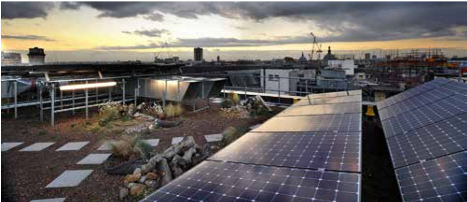
PV panels and green roof combined
