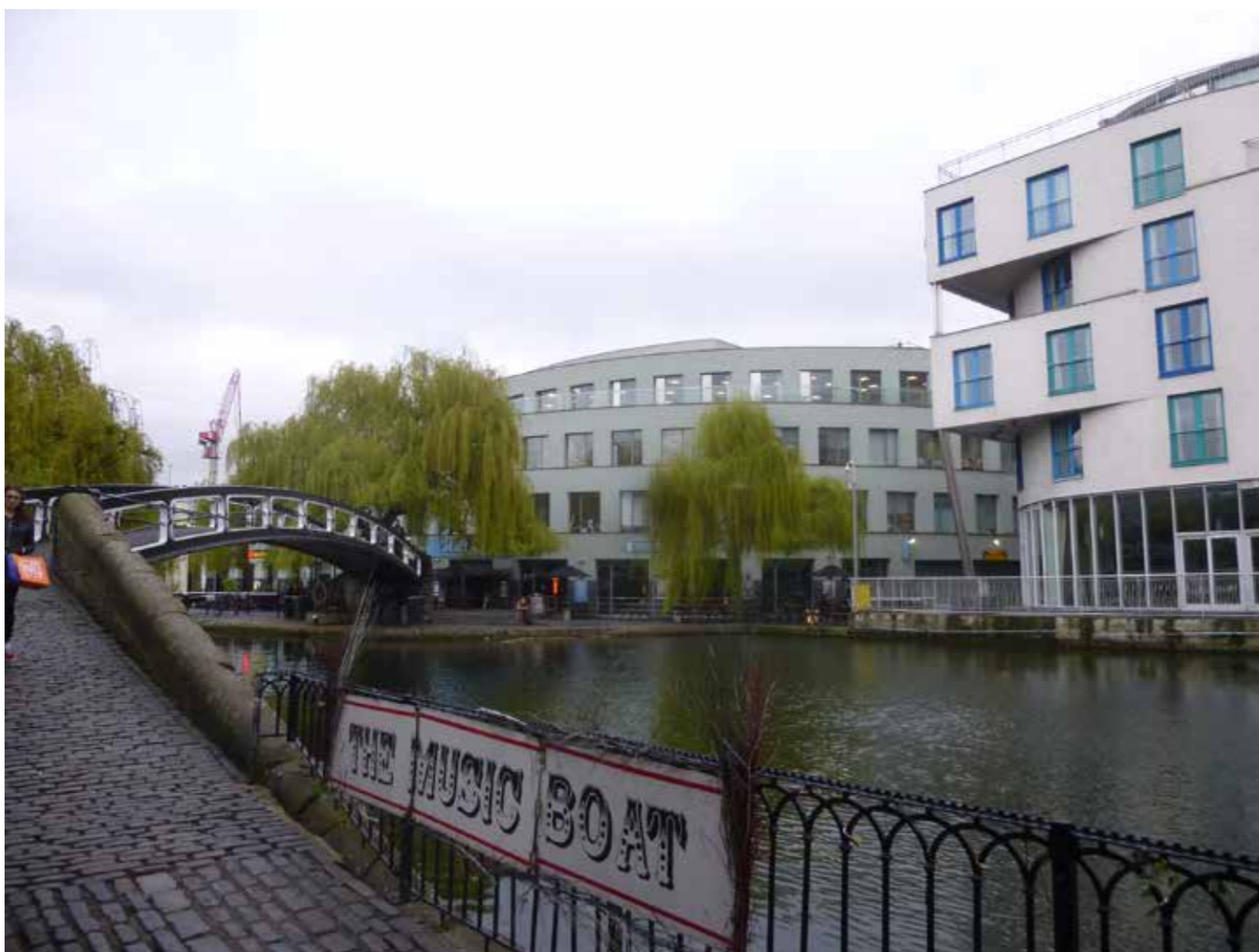
Photograph of the existing building from the other side of Regents Canal
