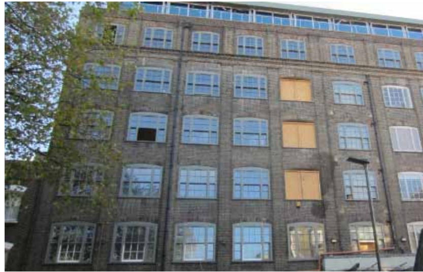
Belmont Street warehouse conversion
