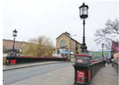
4. Hamstead Road Bridge
