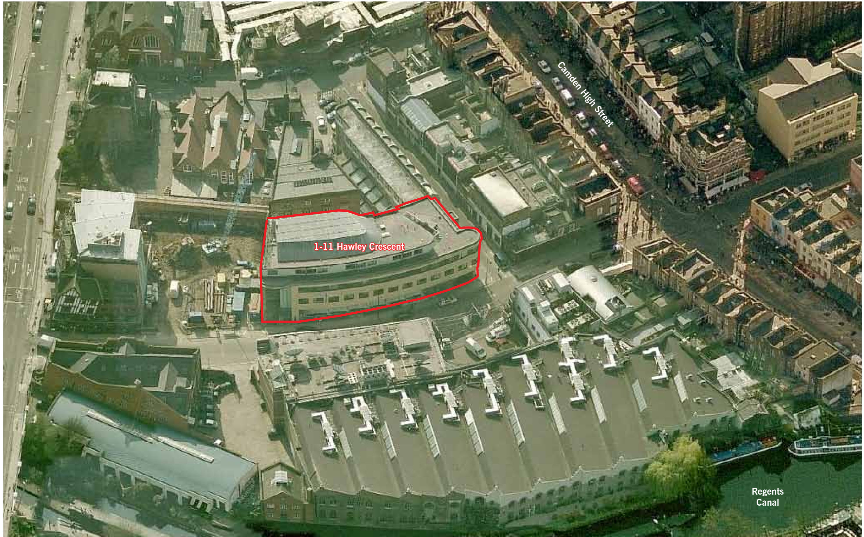
Aerial view showing the application site
