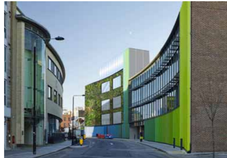
3. Existing view from Hawley Crescent towards the west
