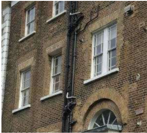
Fig 71: Profusion of pipework
