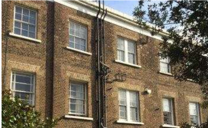
Fig 16: Contrast between window style and lintels
