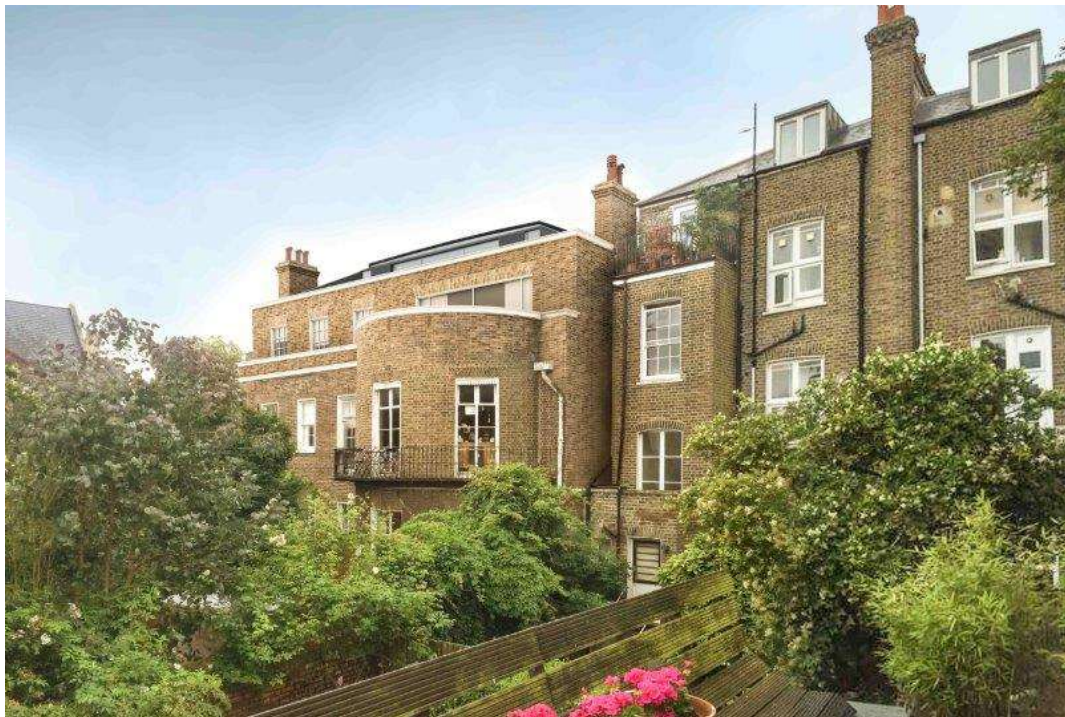
Fig 123: Appearance from view location 7 (note that a higher resolution version of this image is included in drawing 1502-AR-003)
