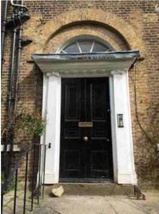
Fig 66: Existing door surround
