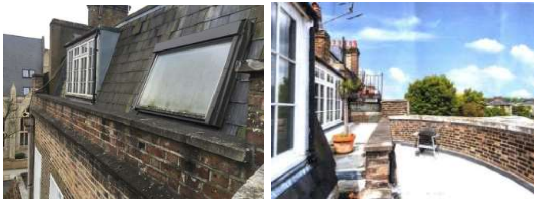
Fig 52 & 53: The rear of Grove End House at second floor level
