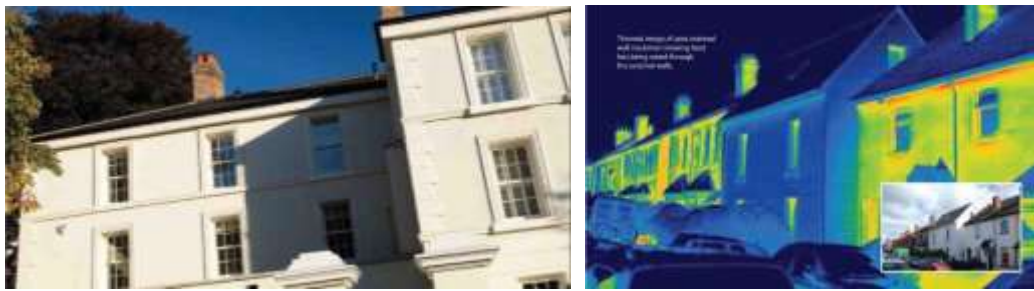
Fig 126 & 127: Externally rendered insulation on a historic building (left) & a thermal image (right)
