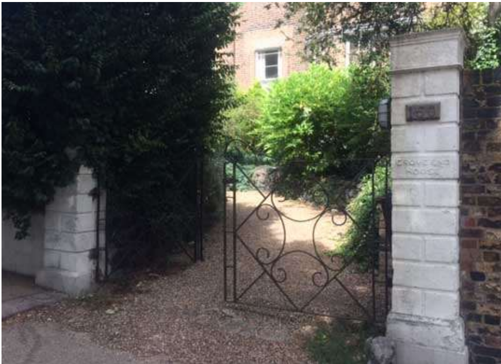
Fig 61: One set of two pairs of gates at the driveway entrances
