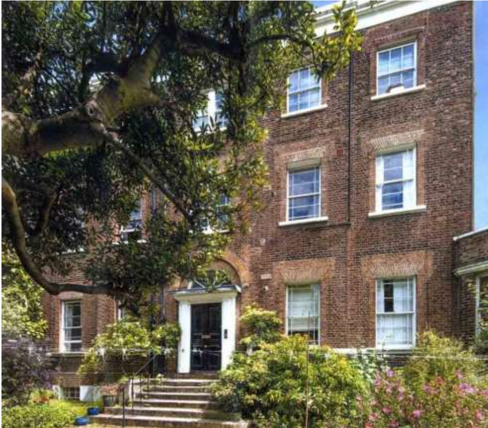
Fig 37: Grove End House front elevation in present day condition
