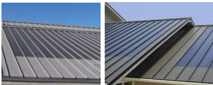
Fig 103 & 104: Examples of thin film photovoltaic systems applied to roofs
