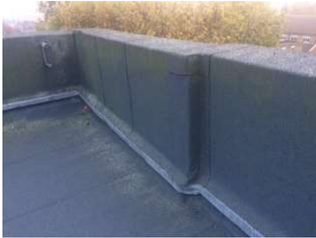
Fig 73: Front parapet showing asphalt lapped onto top
