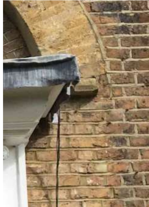
Fig 67: Detail of remains of porch
