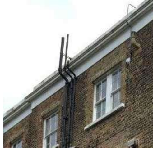
Fig 72: Cranked pipework interrupting cornice
