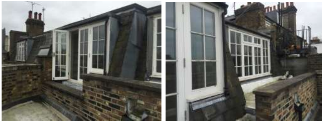
Fig 80 & 81: Uncharacteristic windows on second-floor rear elevation
