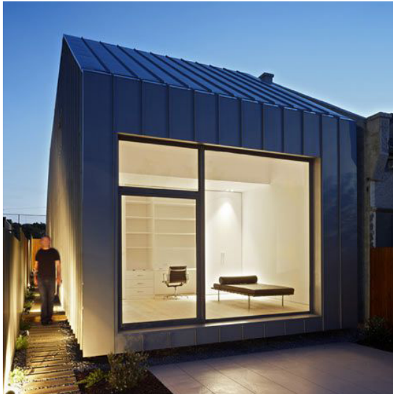
standing seam cladding wrapping from the roof to the wall
