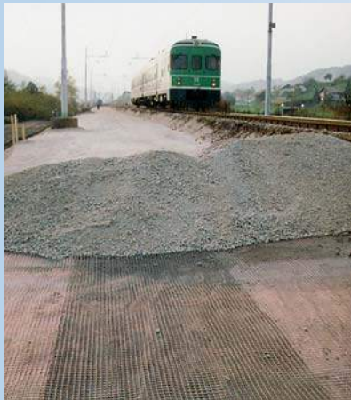
Railroad ballast reinforcement with Tenax LBO geogrids
