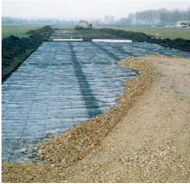
Soft soil stabilisation and separation using Tenax GT.
