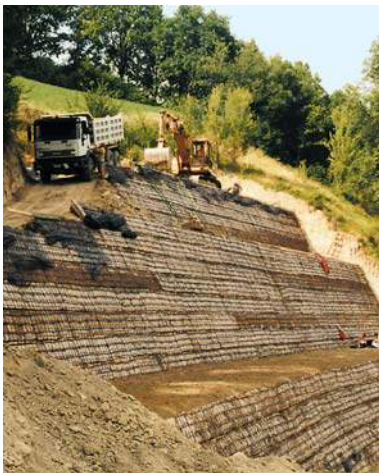
Tenax Rivel system for landslide repair.
